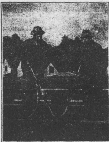
MODERN METHODS OF REPAIRING ROADBEDS
