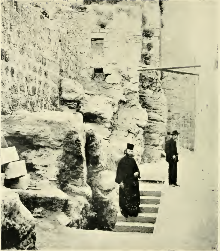
Eastern portion of Rock-scarp.
