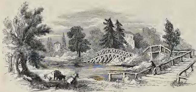
THE WEY BRIDGE.
