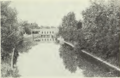
DRAINAGE CANAL toward Sheridan Road bridge.
