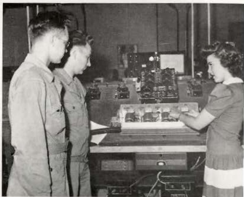
Paralleling of B-17 Engine Generator System.
