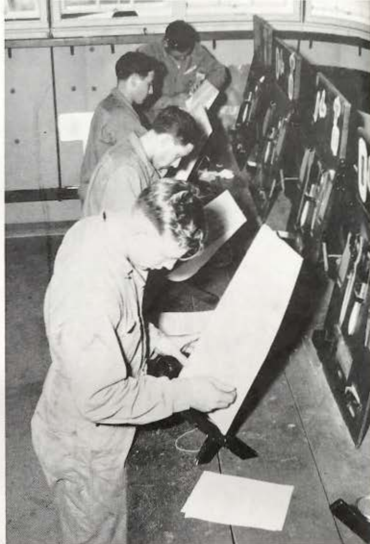
Frame, Fabric Covering and Sewing.
