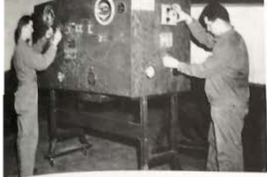
Mockup, Lighting Circuit Wiring.
