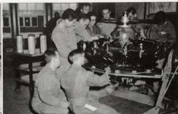
Assembly and Disassembly of Power Sections.
