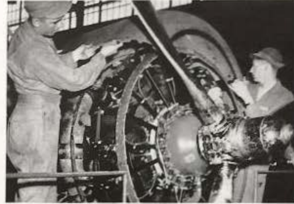
Cowling Installation.
