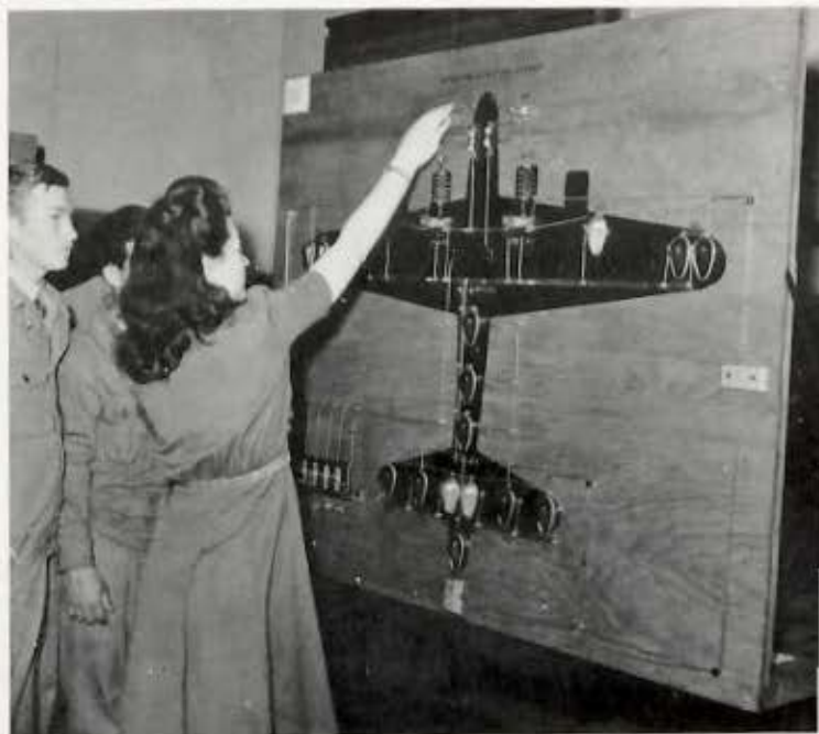
Mockup, Arrangement of Lighting, Ground, Relay, etc., to Show How to Trace Circuits.
