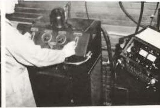
Spark Plug Testing.
