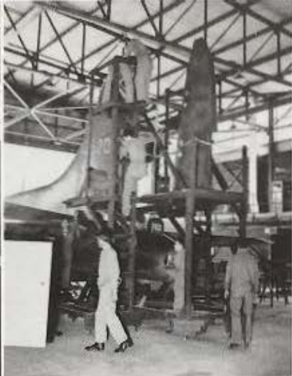
Removing Tail Assembly.
