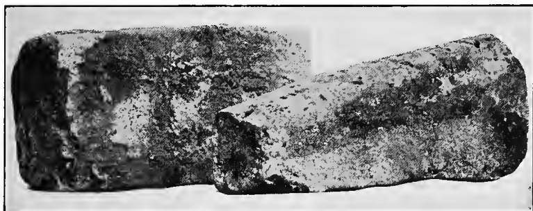
FIG. 143.—Brick from arch and invert of Worcester sewer.
