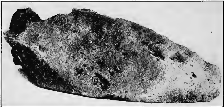
FIG. 145.—Brick from invert of Worcester sewer.
