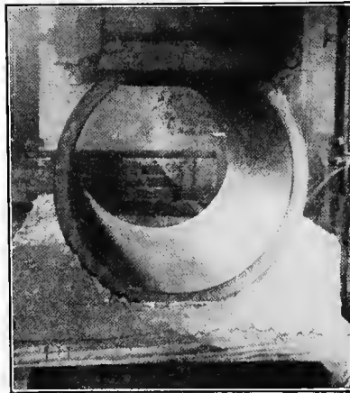
Fig. 109.—Sewer pipe supported in concrete cradle.
