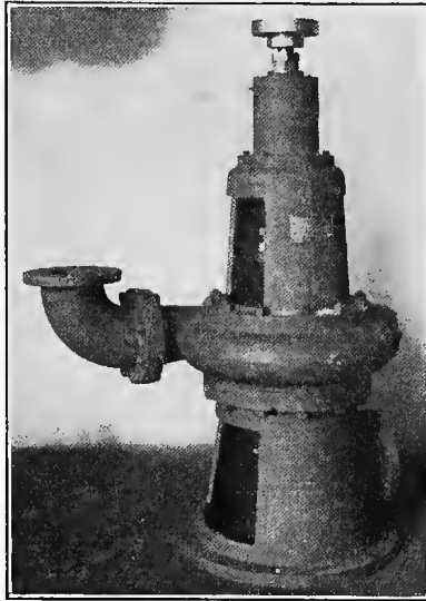
FIG. 270.—Vertical centrifugal pump, single suction, single stage. ( Morris Machine Works. )
