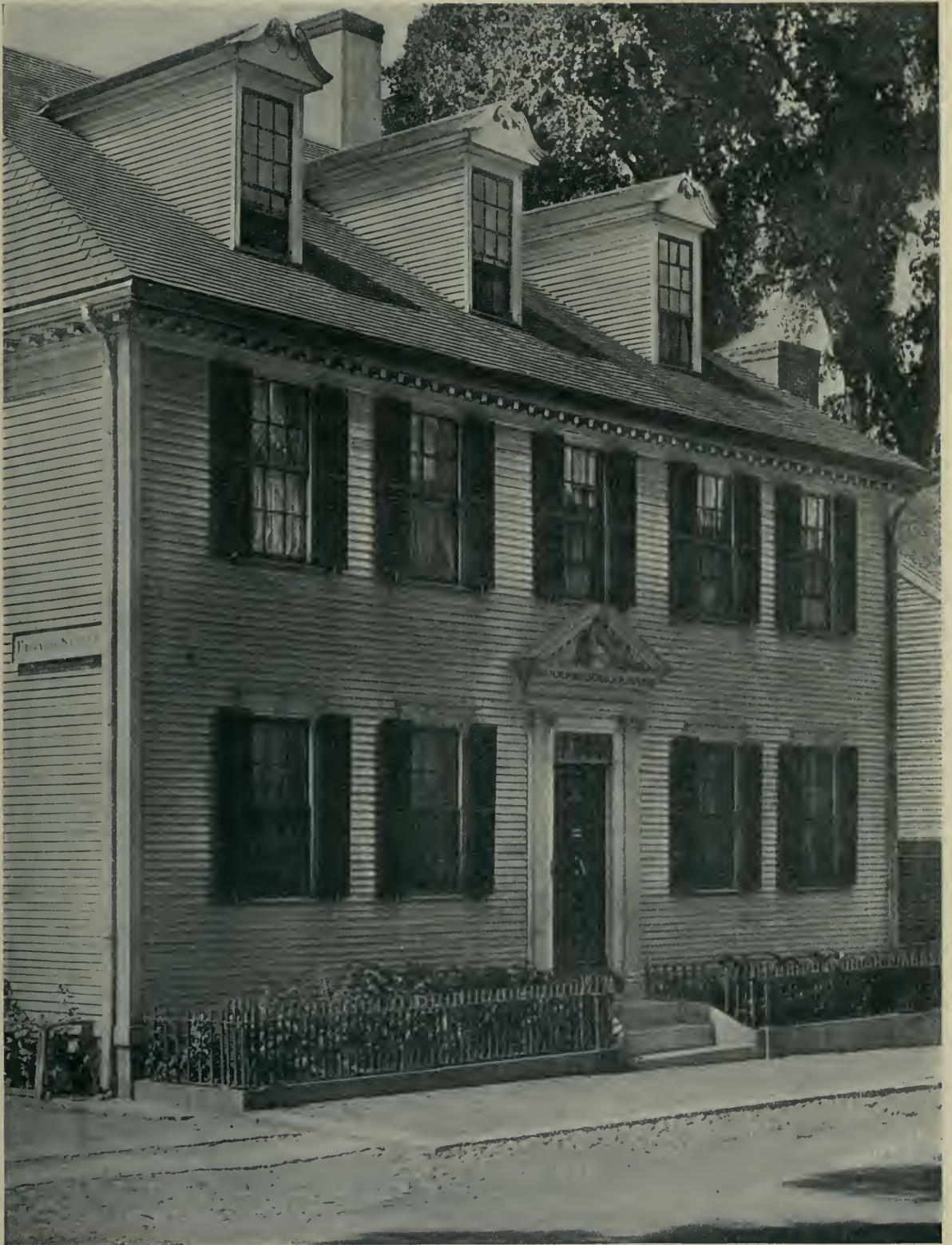
THE JACOB WENDELL HOUSE, PORTSMOUTH, NEW HAMPSHIRE. Built in 1789 by Jeremiah Hill.
