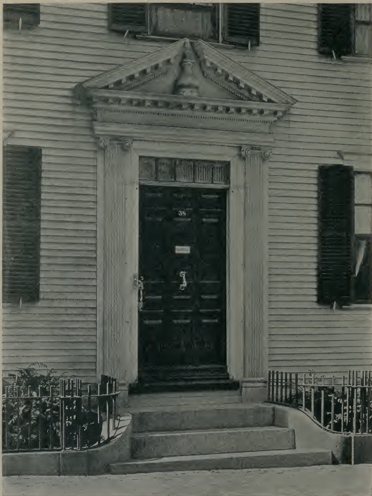
THE JACOB WENDELL HOUSE, PORTSMOUTH, NEW HAMPSHIRE. Entrance Detail—Built in 1789.
