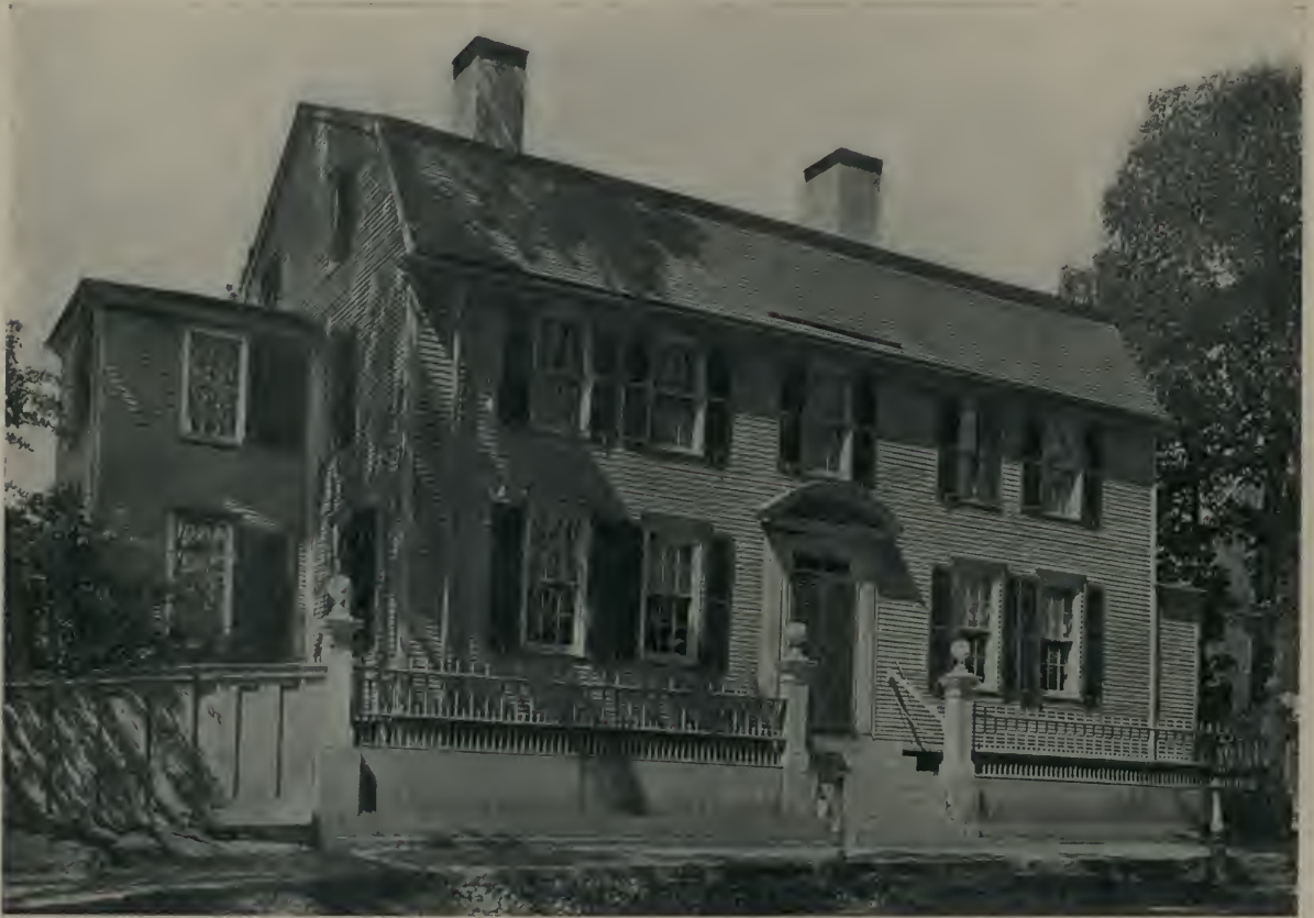
HOUSE AT 124 PLEASANT STREET, PORTSMOUTH, NEW HAMPSHIRE.
