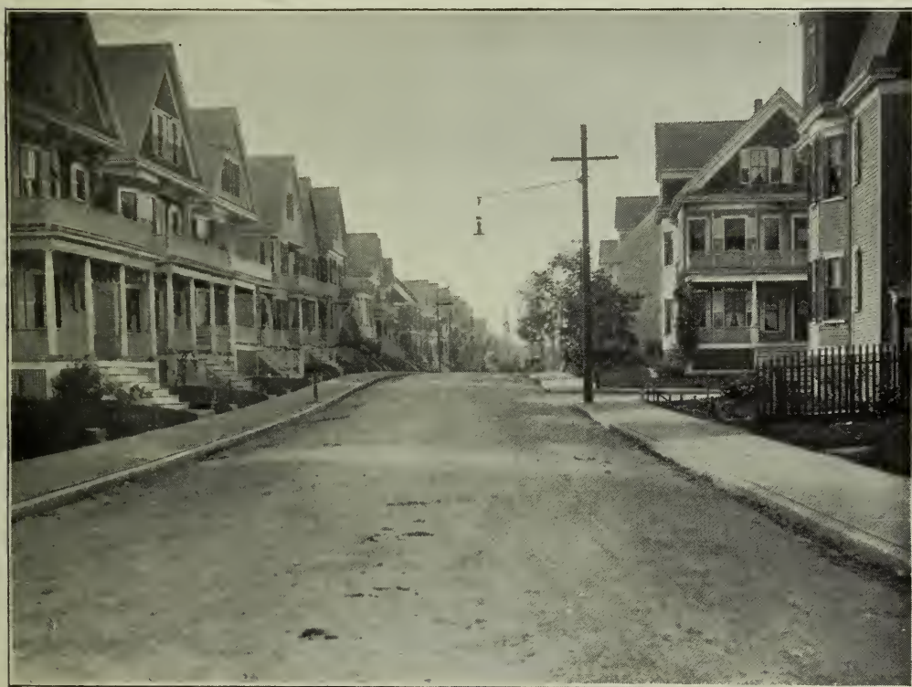
HANCOCK STREET, CONSTRUCTED.
