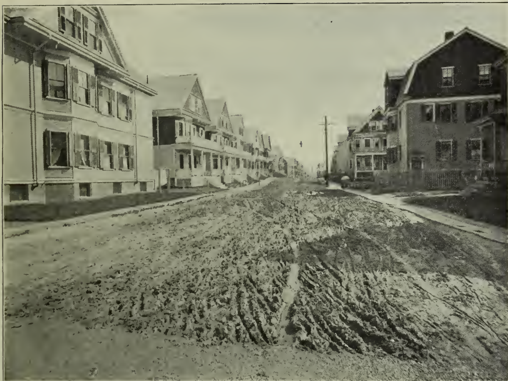
HANCOCK STREET, BEFORE CONSTRUCTION.
