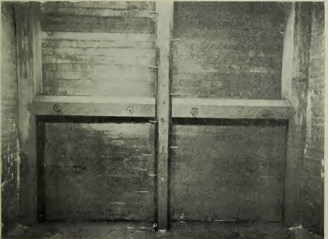
ON STORM DRAIN OUTLET.
