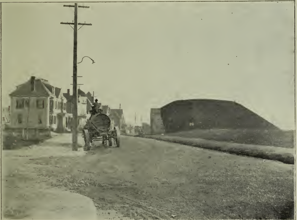
MUNROE STREET, WESTERLY END.
