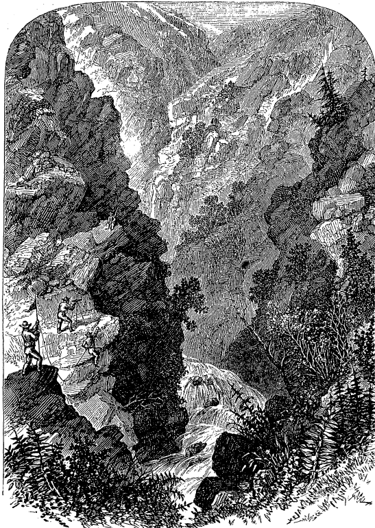
SURVEYING FOR PACIFIC RAILROAD, HUMBOLDT PASS, NEVADA.
