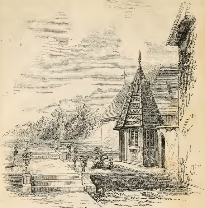
DAIRY, BURNTWOOD GRANGE.
