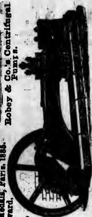
Robey's Improved Horizontal Fixed Engine, fitted with Freely Automatic Expansion Gear.
