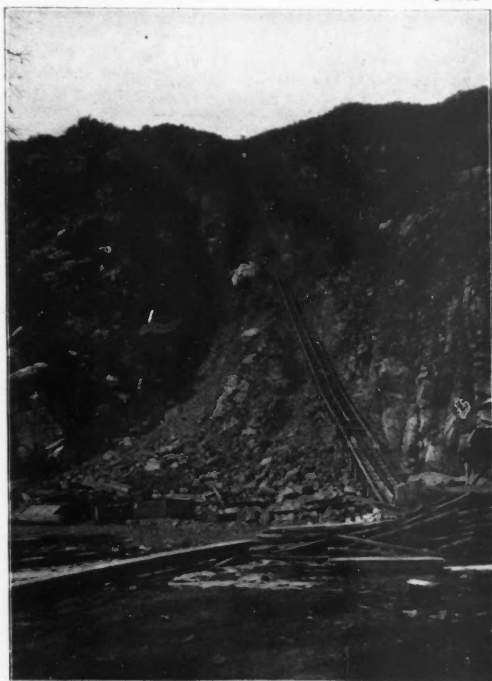
Fig. 7.—Temporary Incline for Hoisting Gravel.
