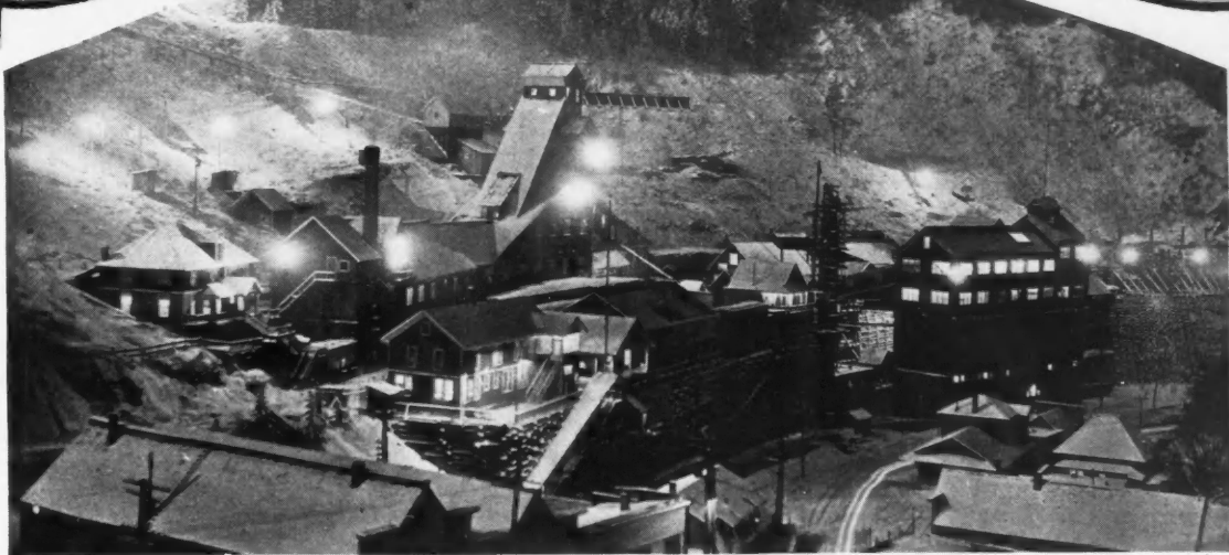
Surface plant of the Hecla Mine, Burke, Idaho, in the Coeur d' Alenes
