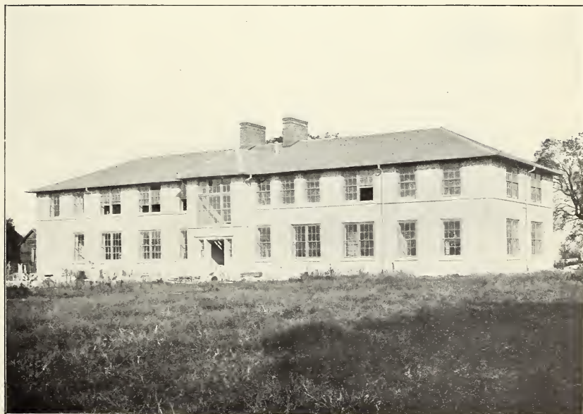
FIG. 2.—DAIRY BUILDING, MISSOURI AGRICULTURAL COLLEGE.
