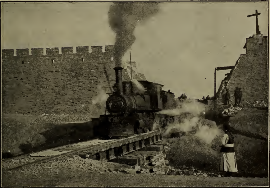
An opening made in the old historic wall of China to admit a railroad into Peking.
