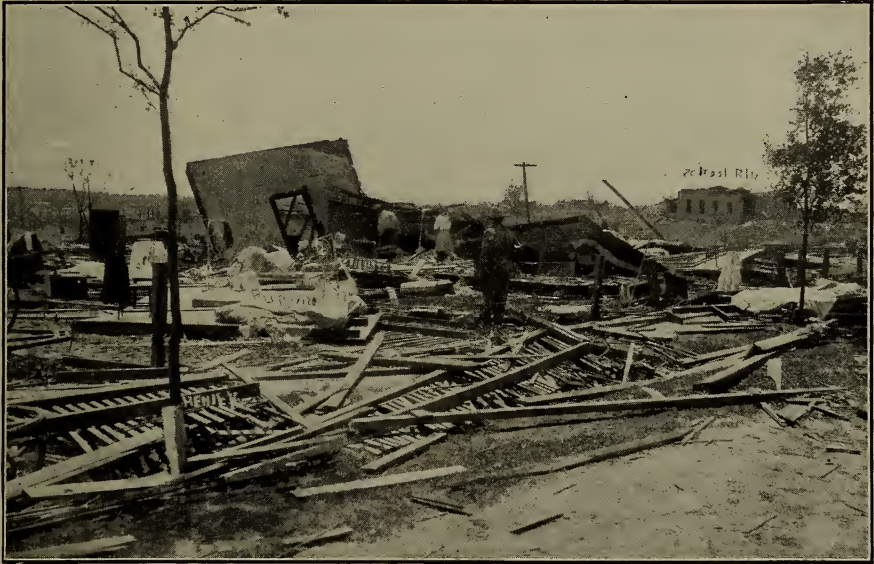
Wreckage in the pathway of the tornado which visited Louisiana, Mississippi, and Alabama, on April 24, 1908. Tornadoes leaving similar destruction in their track during 1908 visited Texas, Oklahoma, Minnesota, Nebraska, Kansas, New Mexico, Iowa, Portugal, and Hungary.
