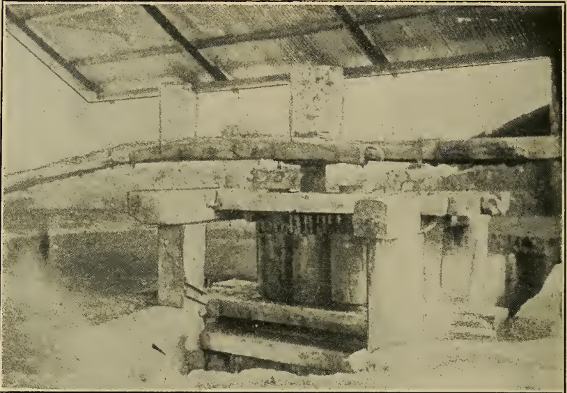
FIG. 3.—Sugar rolls made of copper and operated by animal power. They are claimed to have been introduced by the Spaniards at the time of the Conquest.
