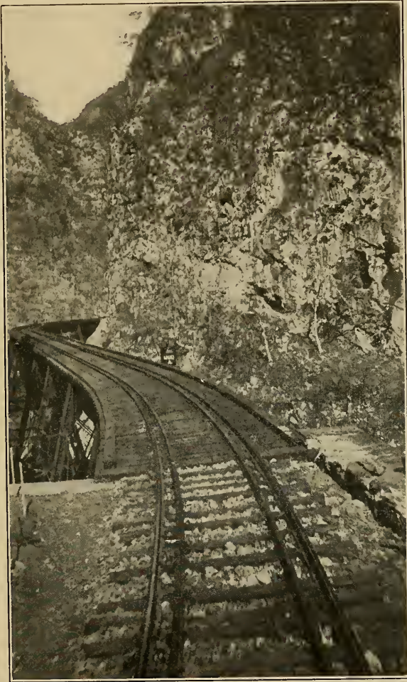
FIG. 4.—Curved steel trestle in a cañon on the Cuernavaca Division of the Mexican Central Railroad.
