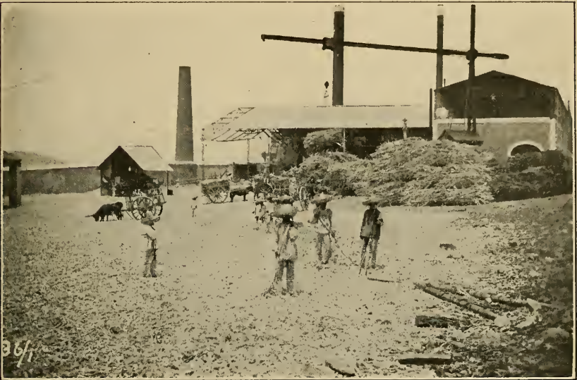
FIG. 7.—Interior of a sugar hacienda in the State of Morelos, Mexico, showing sugar-cane being handled from ox-carts by steam derricks, and in the foreground bagasse drying for use as fuel.
