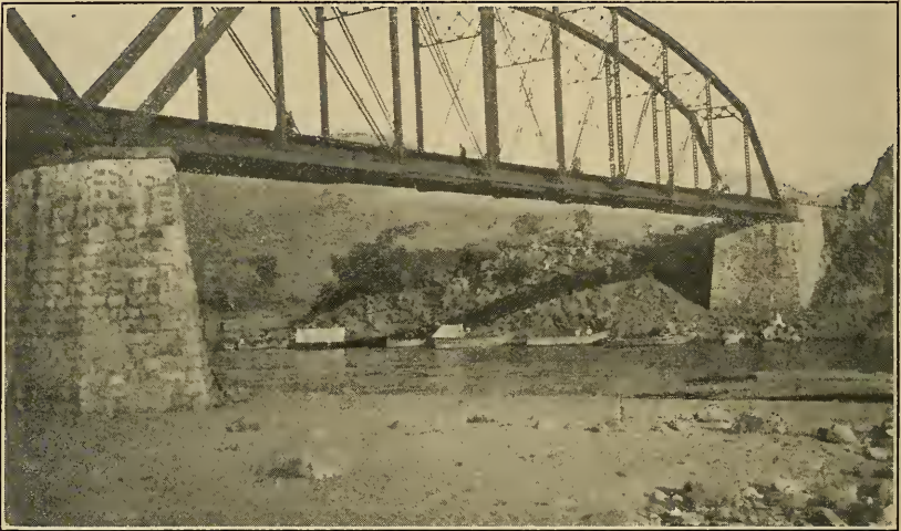
FIG. 3.—One span of a steel truss railway bridge at Balsas, Guerrero, forming the terminus of the Cuernavaca Division of the Mexican Central Railroad. The flat boats shown are utilized to convey freight down the Rio Balsas to various settlements and mining centers.
