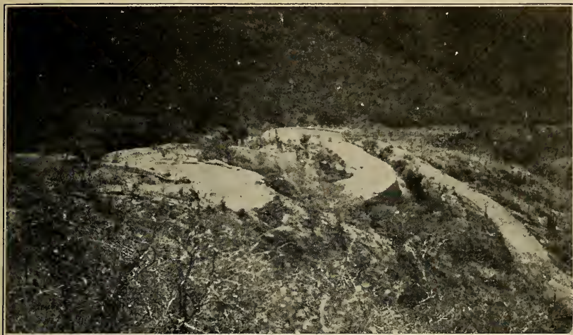
FIG. 10.—Wagon road ascending mountain face near Acatlan, Puebla; average grade about ten per cent.
