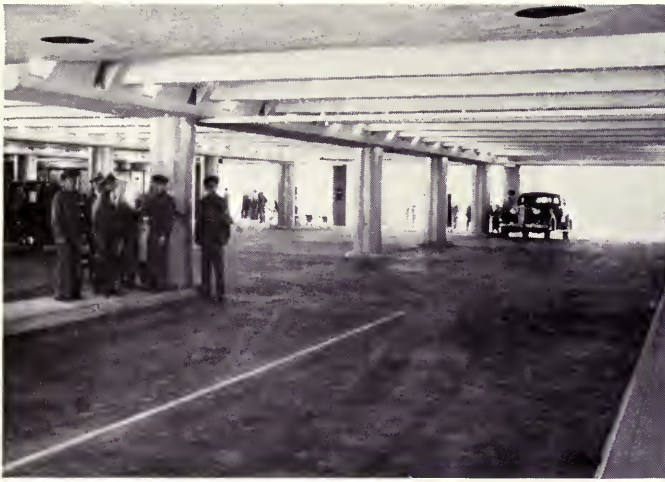
ROCKEFELLER CENTER PARKING—1940. SIX FLOORS IN NEWEST 16-STORY BUILDING
