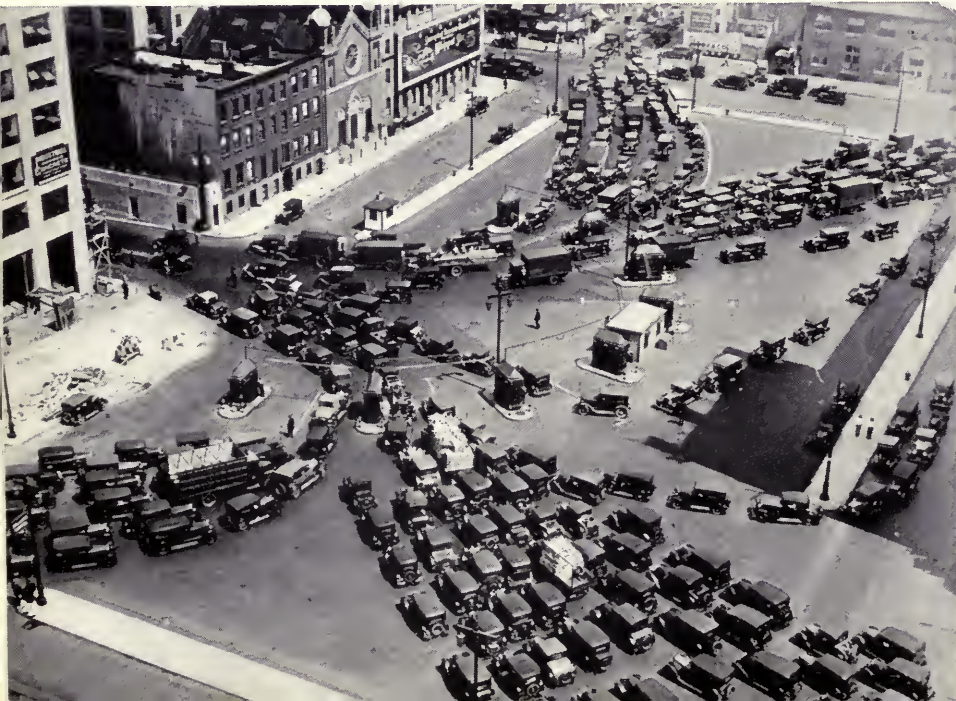
Port of New York Authority
