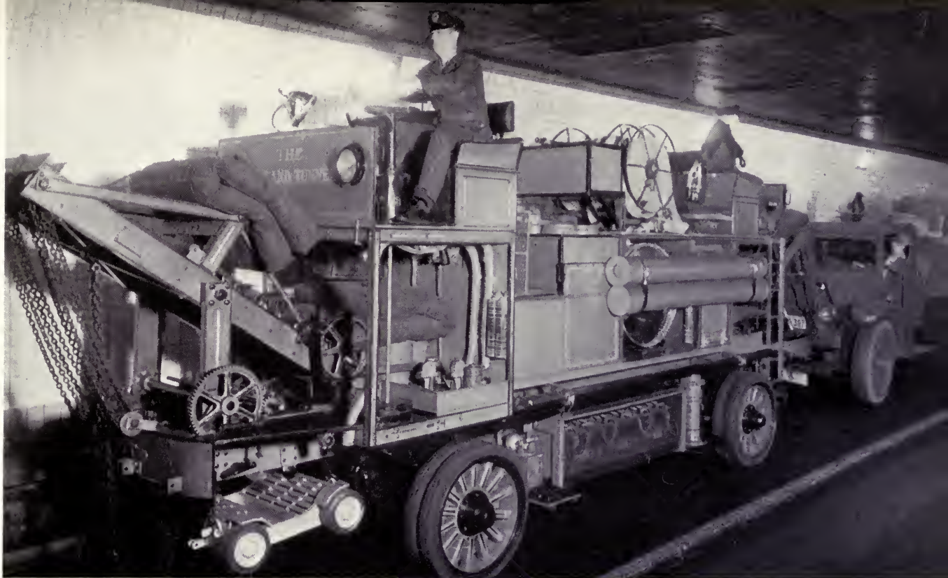
Port of New York Authority
