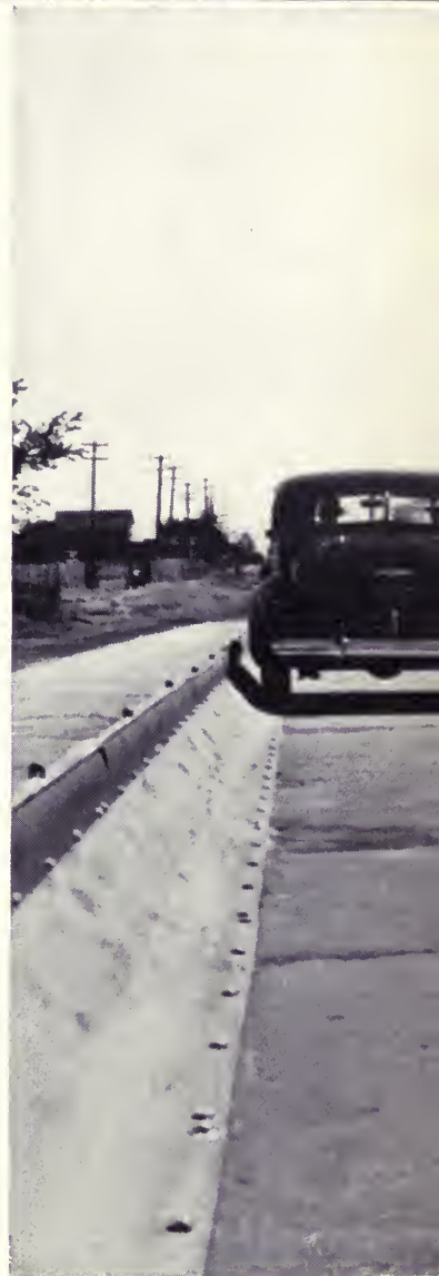
METAL ADAPTATION OF SIDE BARRIER
