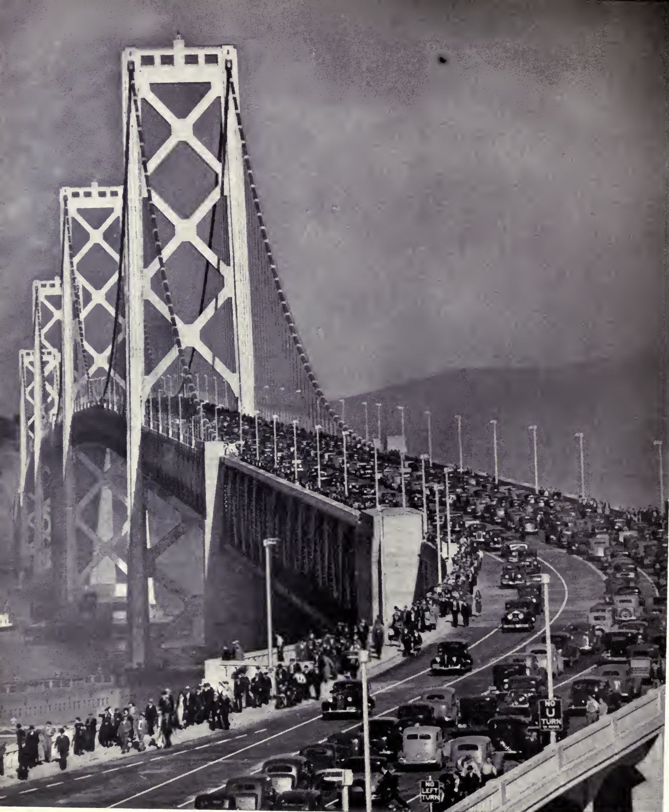
BAY BRIDGE, SAN FRANCISCO
