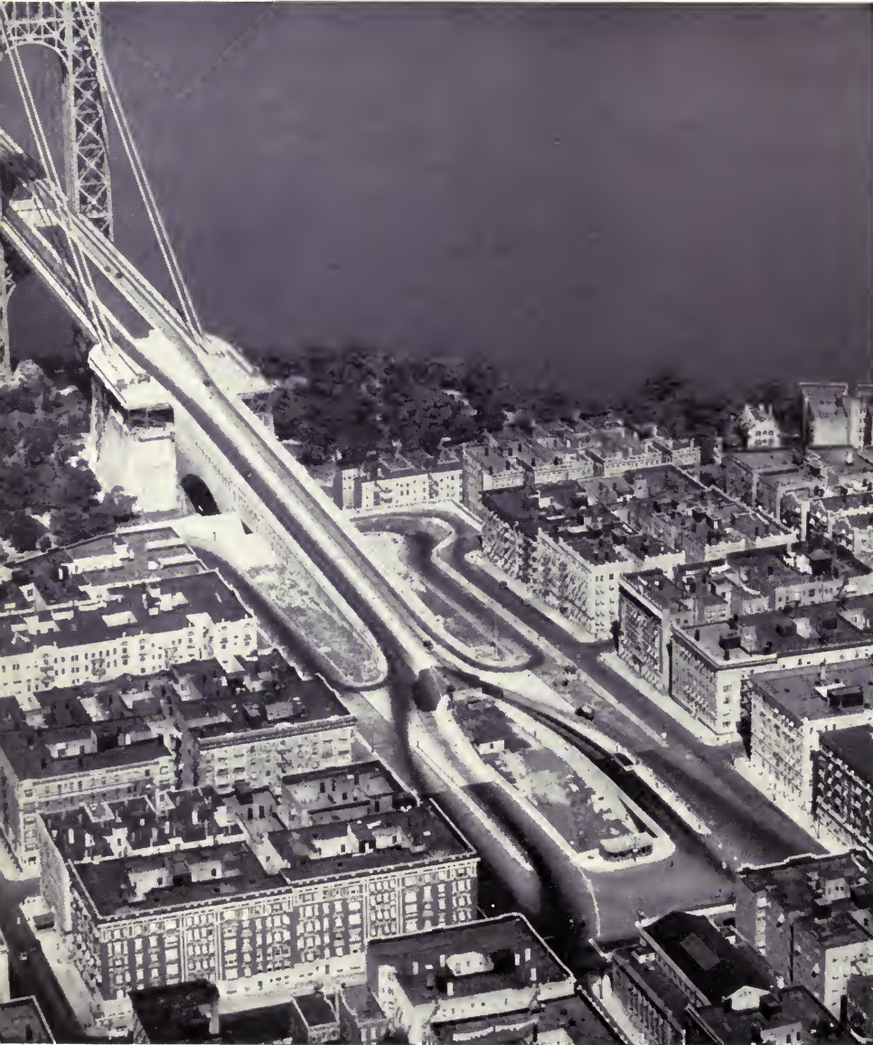
APPROACH TO NEW YORK'S GEORGE WASHINGTON BRIDGE
