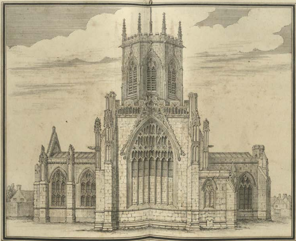
EAST VIEW OF NANTWICH CHURCH.
