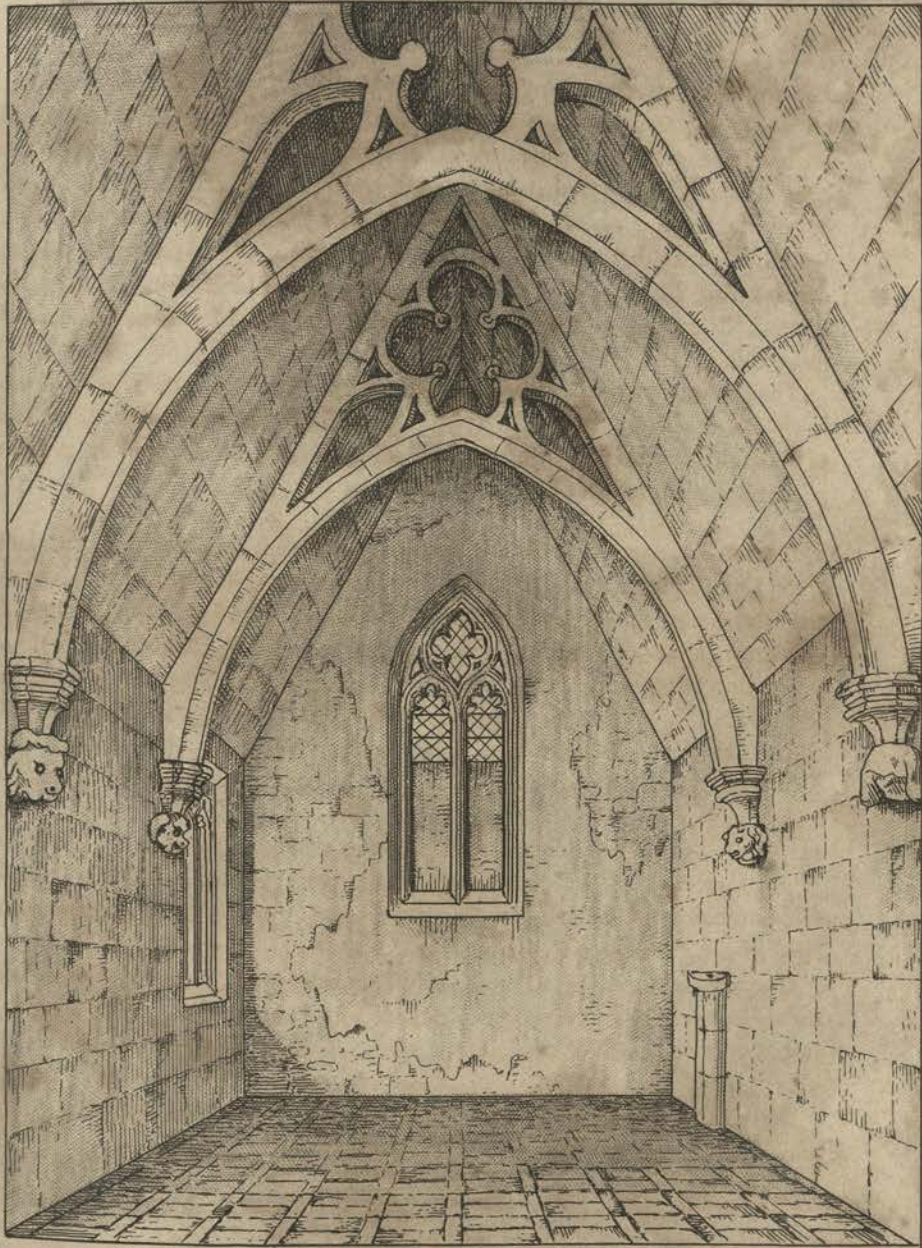
Chapel adjoining the Chancel of Willingham Church.
