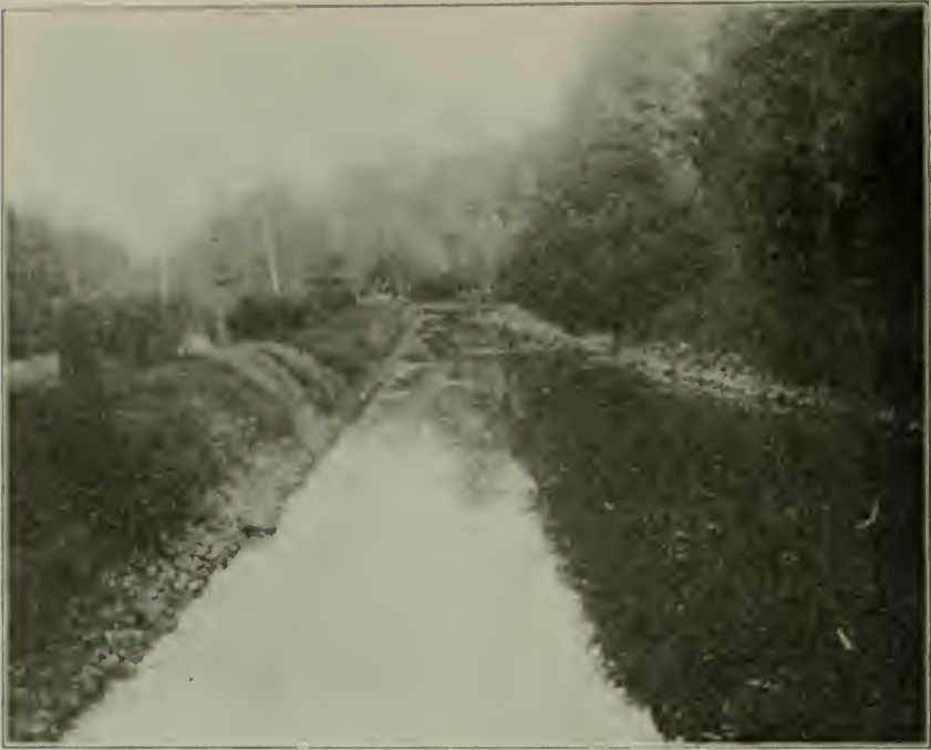
London Water System. No. 1—Pond East of Pump House.
