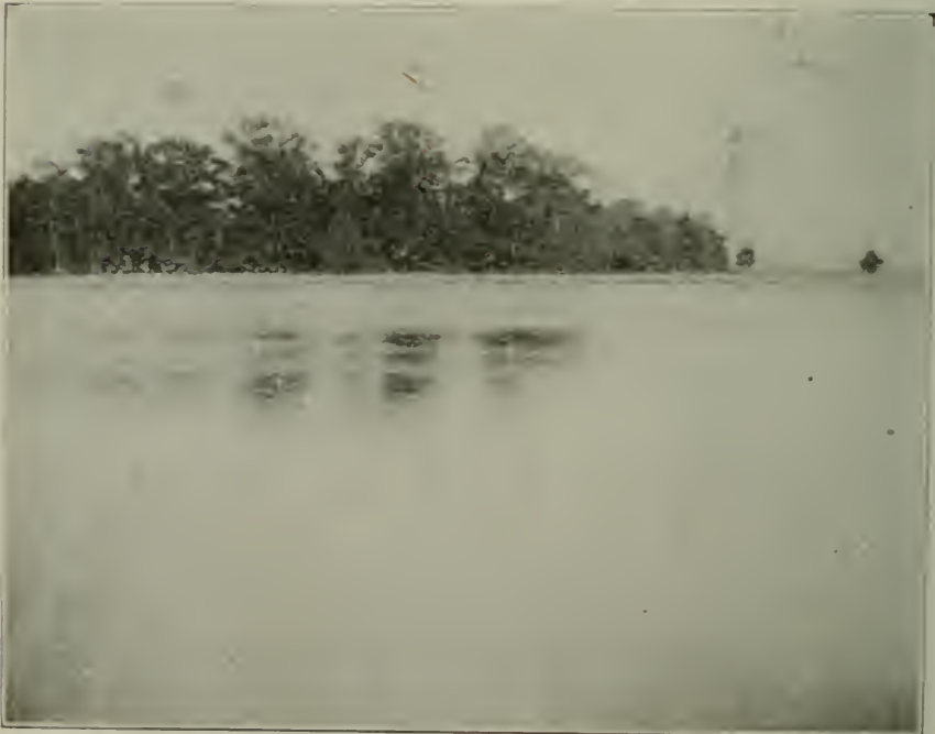
London Water System. No. 4—The Reservoir.
