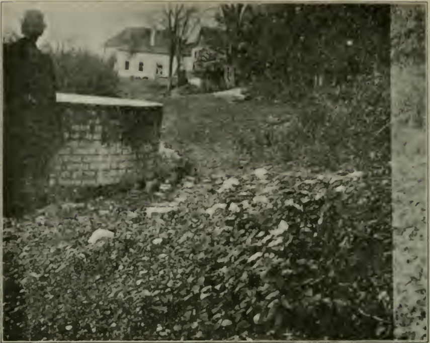
London Water System. No. 5—Showing the Wells and Pump House.
