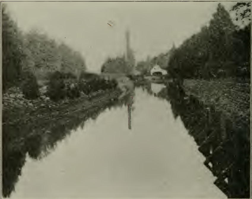
London Water System. No. 2—Pump House and Pond to the West.
