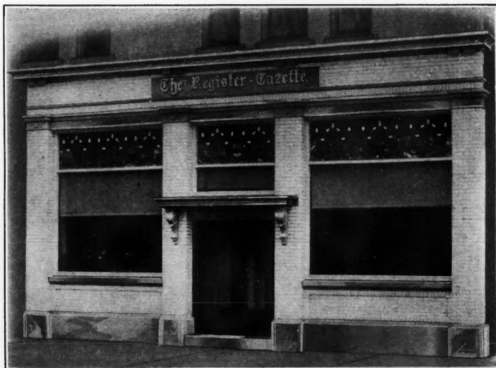
NEW BUILDING OF ROCKFORD (ILL.) REGISTER-GAZETTE.
