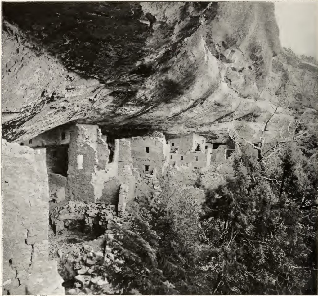
SPRUCE TREE HOUSE HIDES UNDER A HUGE OVERHANGING CLIFF
