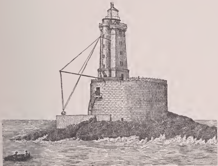
FIG. 5.—Northwest Seal Rock lighthouse.
