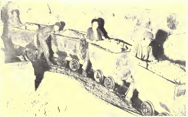
TRUCKING THE ORE TO THE SHAFT
