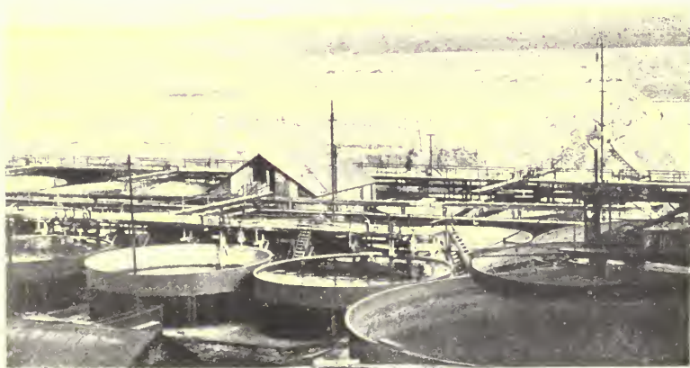
VIEW OF CYANIDE WORKS
