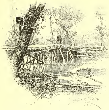
WOODBURY'S BRIDGE ACROSS THE CHICKAHOMINY (SEE NEXT PAGE). FROM A WAR-TIME PHOTOGRAPH.
