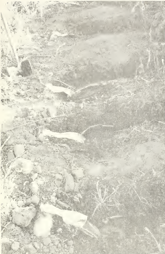
Figure 16.--Outlets in a high pressure section of the Kemper installation, with and without energy dissipators.
