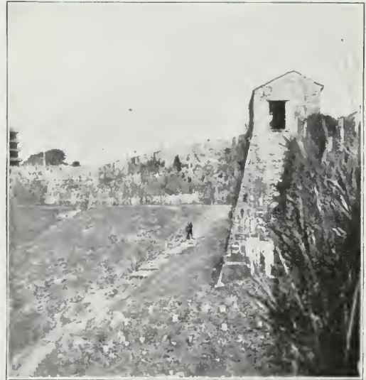
Old Wall, Canton (now demolished)
