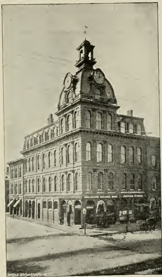
Mechanicks' National and Merrimack County Savings Bank
