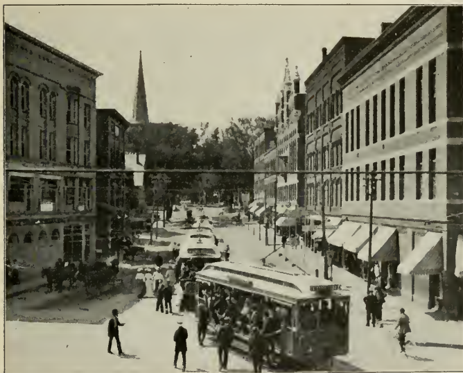
Looking Up Pleasant Street
