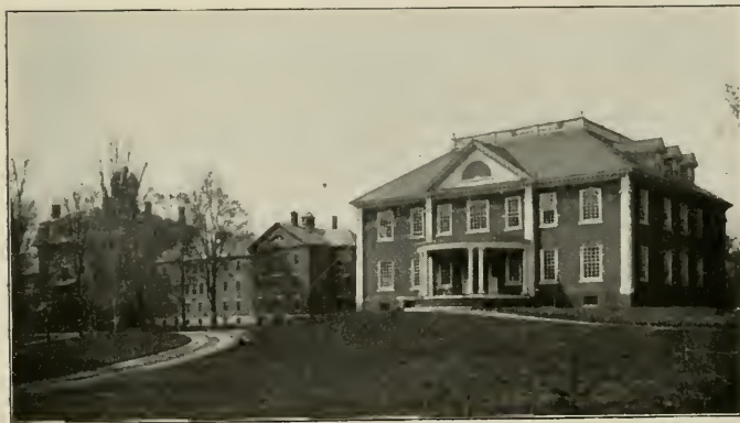
State Hospital Buildings
