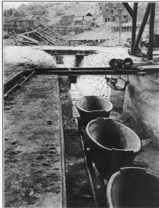
MOVABLE LAUNDER PREVENTS SPILLING WHEN FILLING MATTE LADLES
