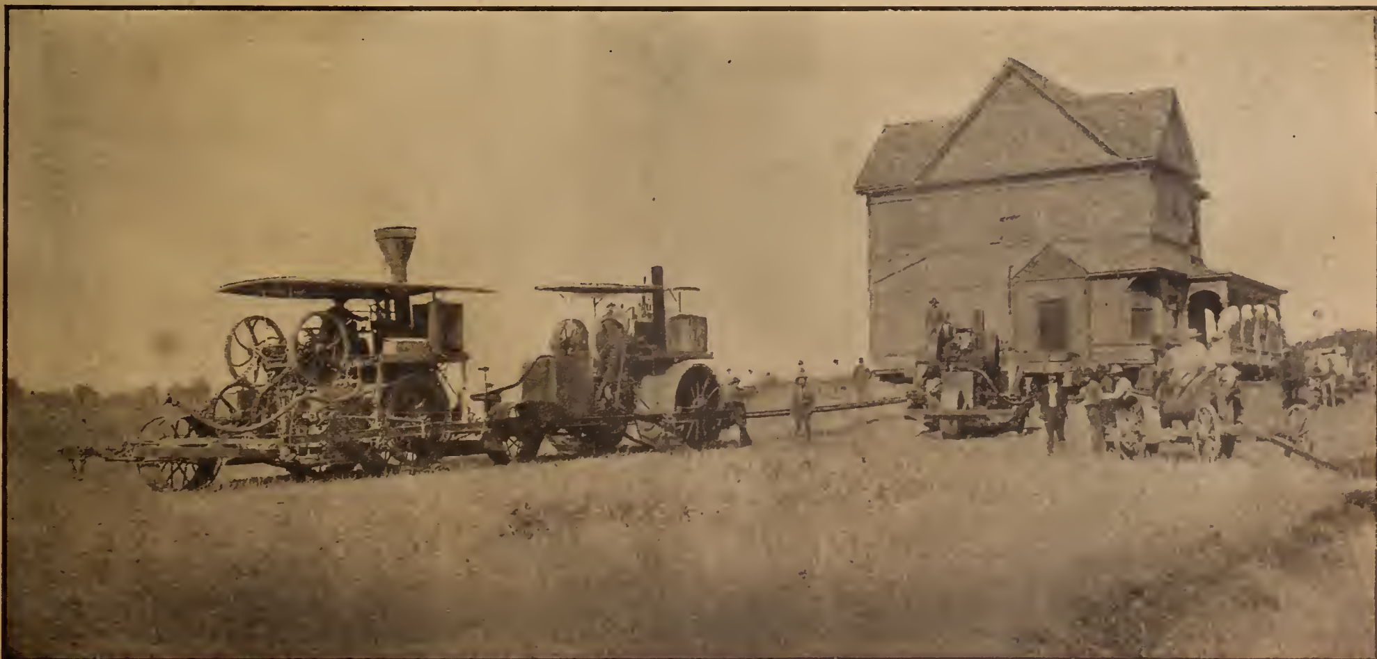
MOVING A FARM HOUSE OVER FIELDS BY MEANS OF TRACTION ENGINES
