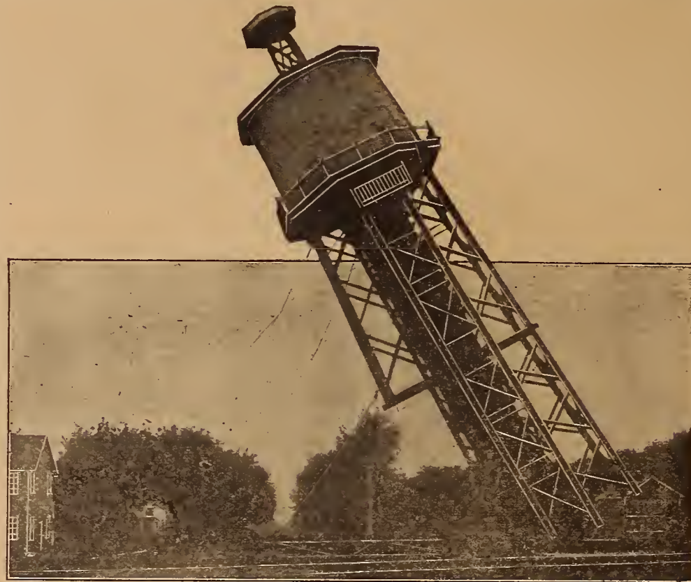
WRECKING AN OLD WATER TOWER
