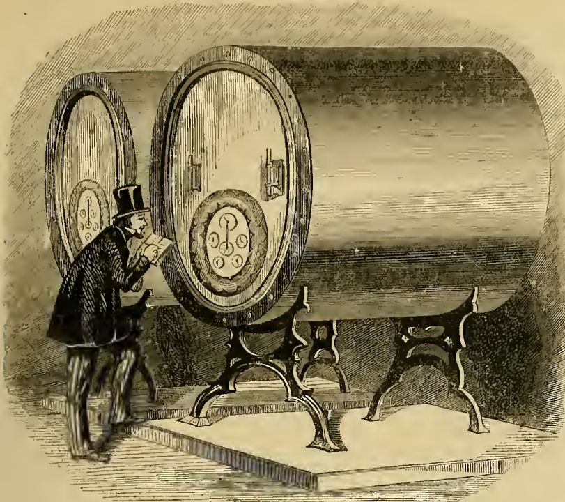
THE METRE ROOM IN THE PHILADELPHIA GAS WORKS.
