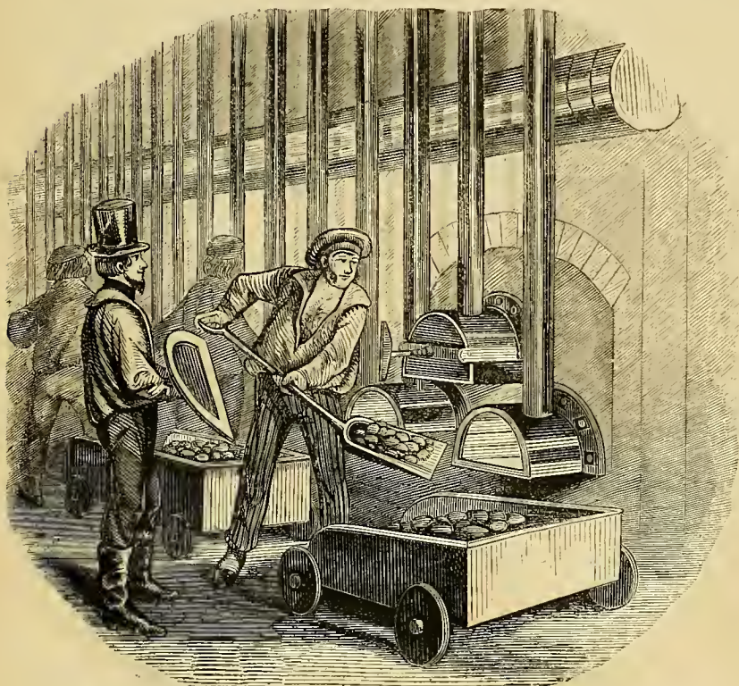
THE RETORT ROOM IN THE PHILADELPHIA GAS WORKS.
