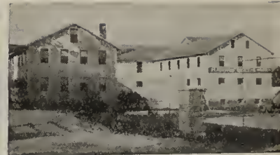
Office and Main Warehouse
