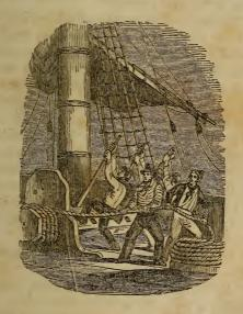
"The pulley, as you know, is a wheel with a groove, or hollow, round it; this is fixed in a block of wood. If a cord be passed over the pulley, it enables a man to lift a weight with much greater ease than he otherwise could do; and if he made use of several pulleys, a still greater weight might be lifted. The greater the number of the pulleys, the easier is the weight removed."
