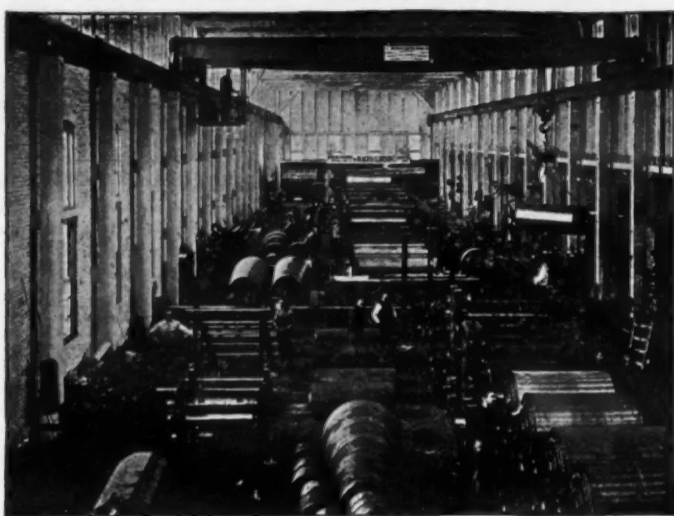
Erecting Department of the Black & Clawson Co. Shops, 50 ft. x 270 ft.
