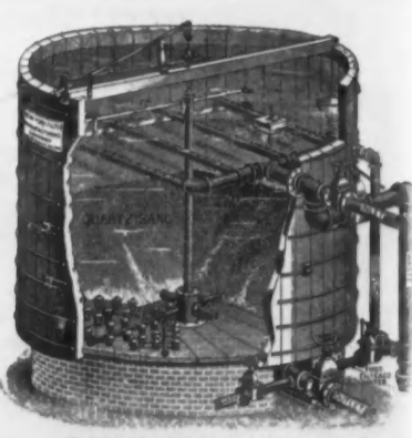
NEW YORK TYPE GRAVITY FILTER.
