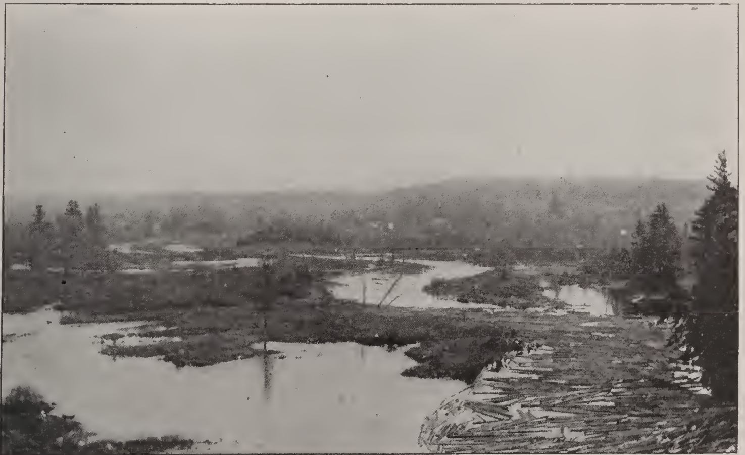
PROPOSED HARRISVILLE RESERVOIR. Lower End of Basin.
