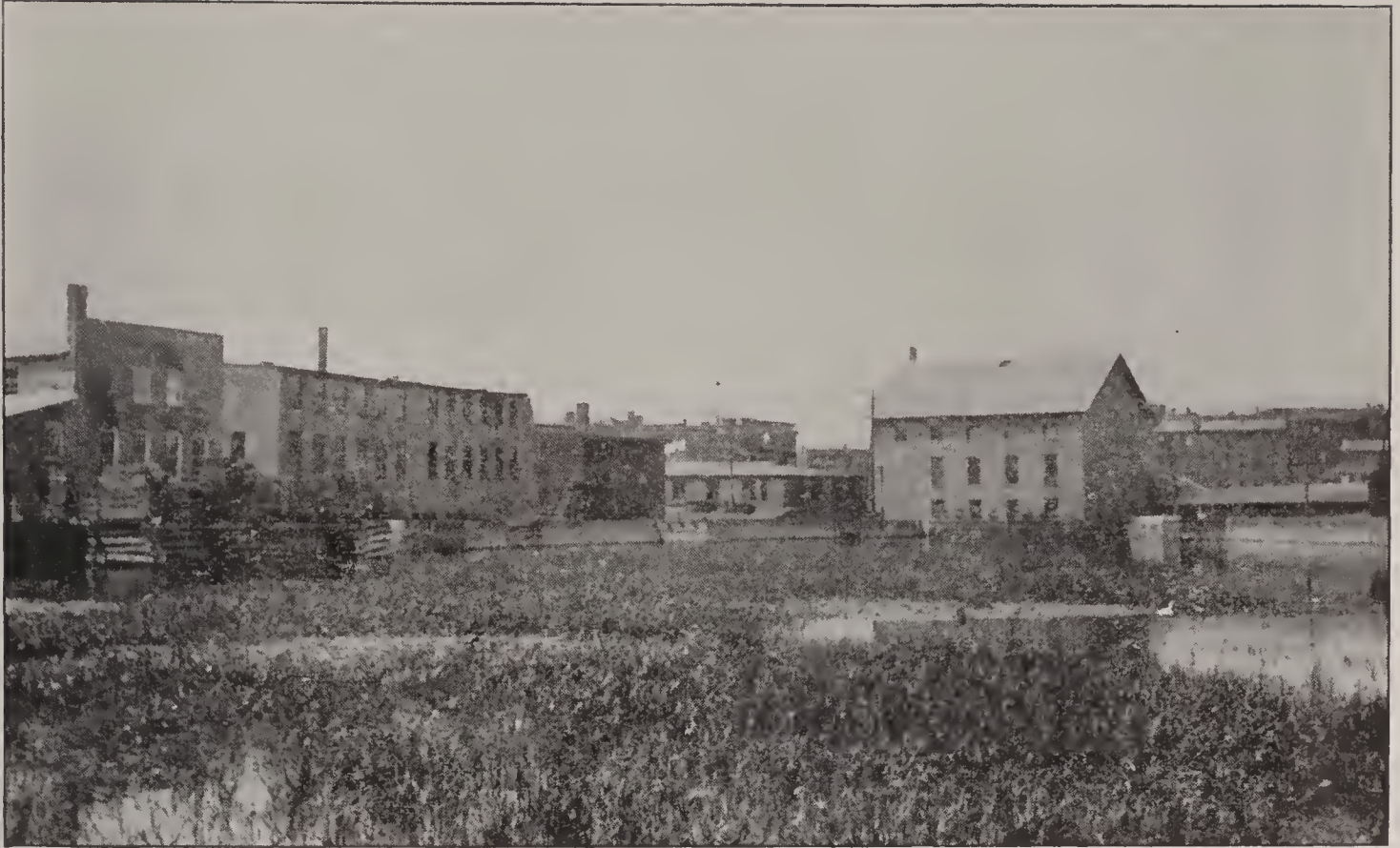
END OF POWER CANAL OR "BASIN" AT OGDENSBURG. Filled with Mud and Overgrown with Water Plants.
