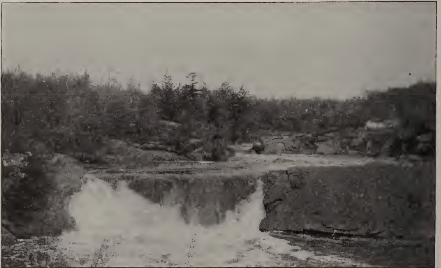
ROCK DAM — INCLUDED IN MADISON CHUTE POWER PROJECT.
