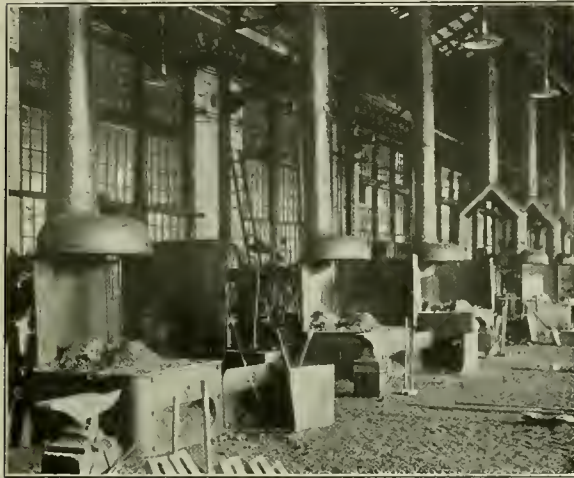
Fig. 5—Blacksmith Shop, Showing the Arrangement of the Lights
