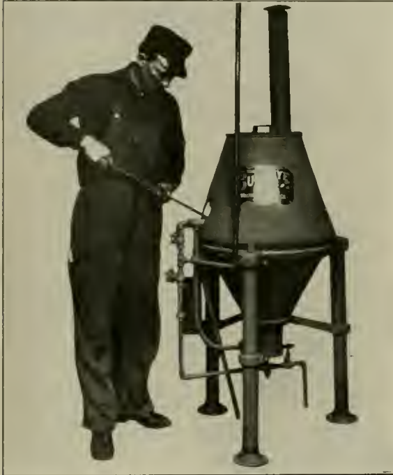
Files Being Cleaned in a Buckeye Machine
