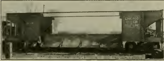
Fig. 1—Side Dump Car Being Stripped for Repairs
