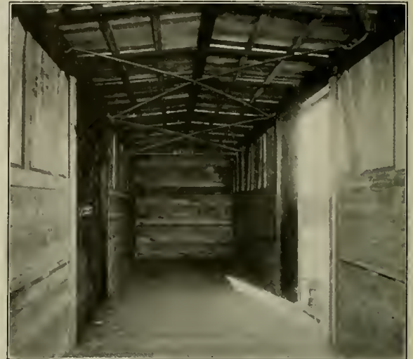
Fig. 5—Interior View of Strengthened Furniture Car Showing the Roof Bracing
