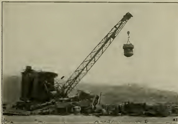
Locomotive Crane Breaking Large Scrapped Castings
