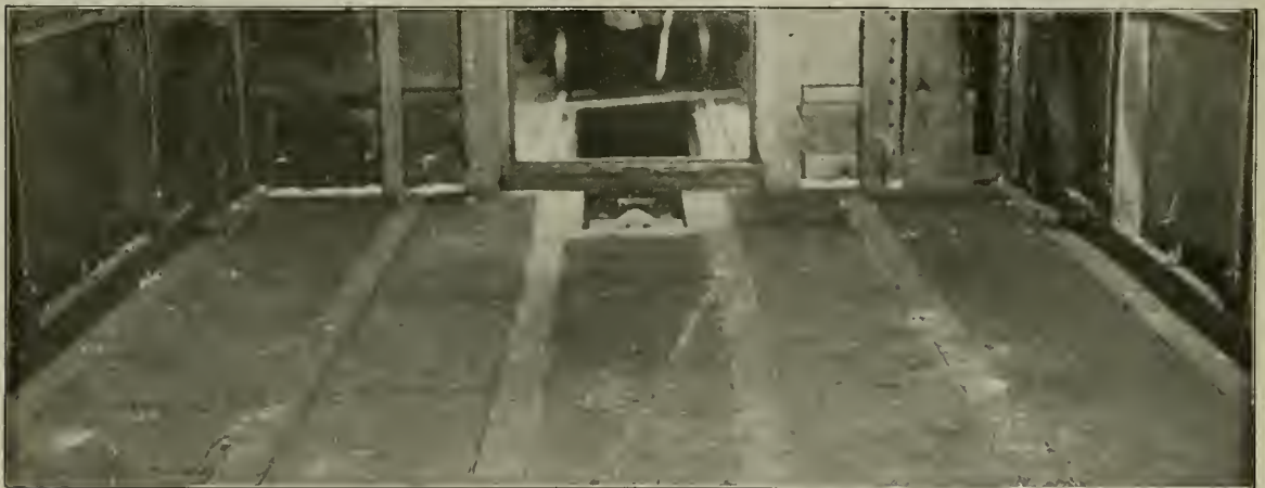
Tucork Floor Insulation in Place
