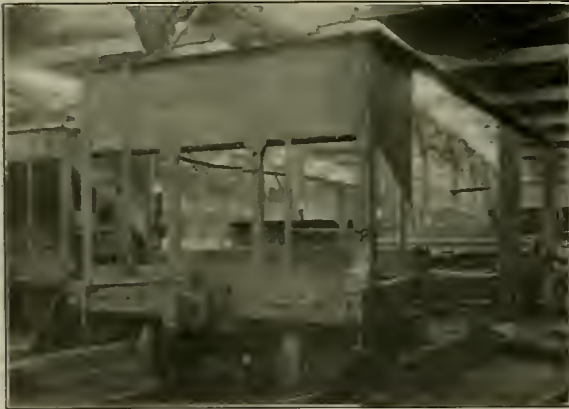
Fig. 2—Bottom Dump Car Ready for the Application of New Sheets
