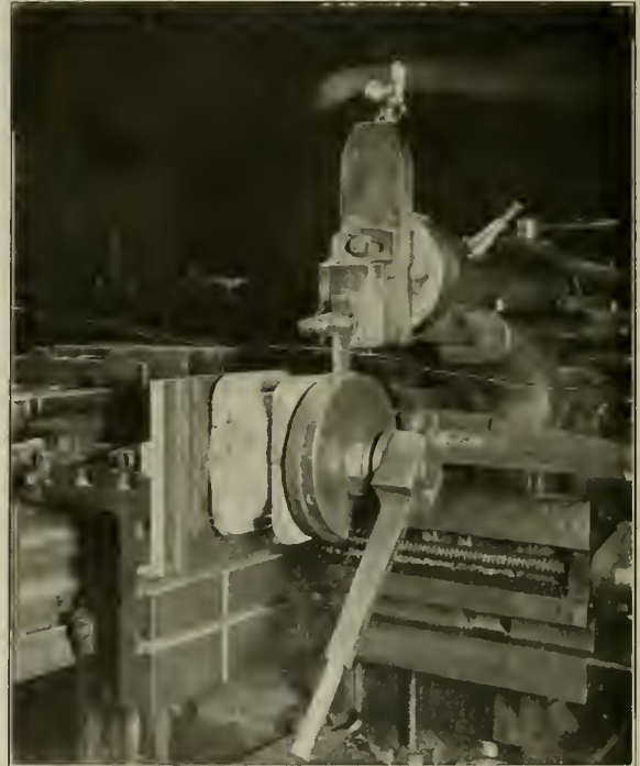
Shaping the Strap Fit on Main Rod Brasses
