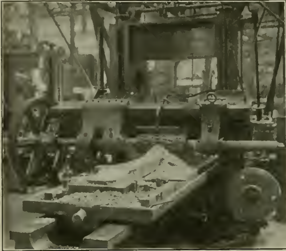
Fig. 5—Finishing the Sides of a Rod on a Slab Milling Machine
