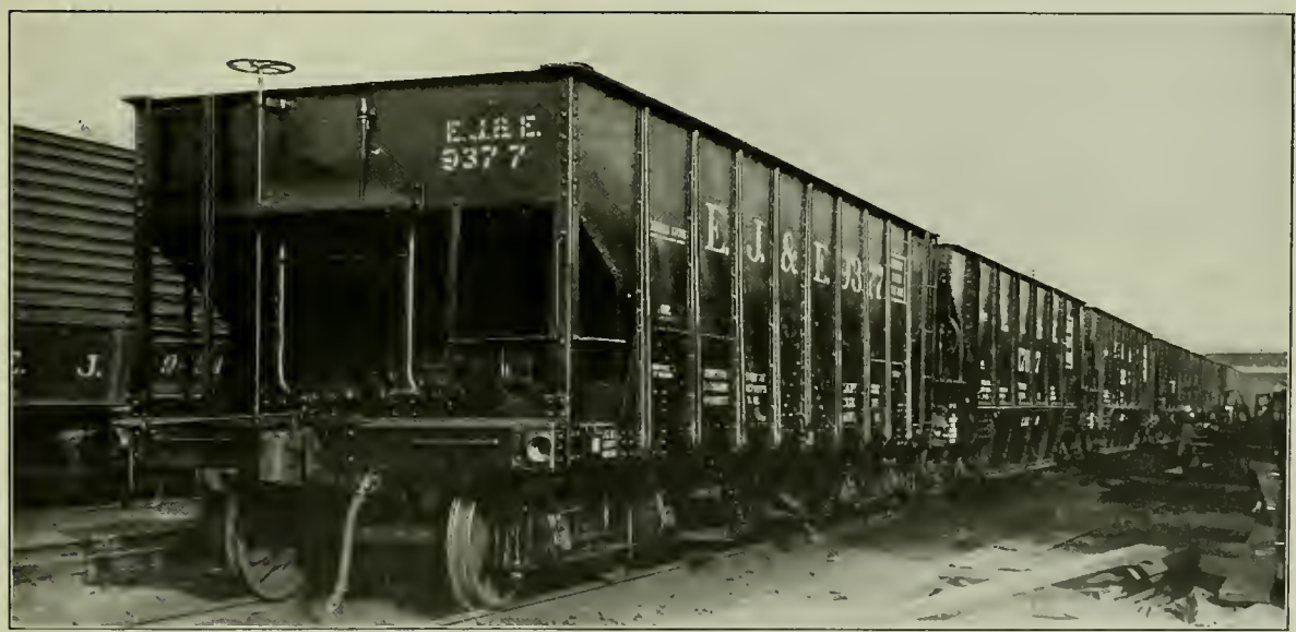
The Day's Output Ready to Leave the Repair Track
