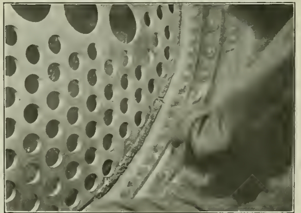
Welding a Front Tube Sheet
