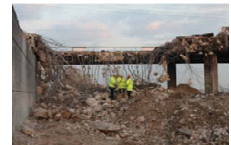
Bridge demolition after the fire incident
