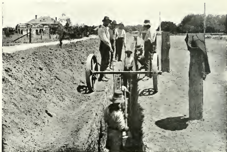
Laying 18 inch "Pioneer" Wood Pipe Mildura Irrigation Trust.
