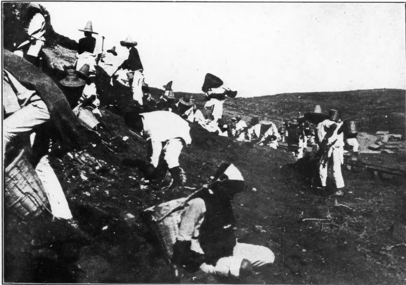
EXCAVATING FOR PINGUICO MILL, GUANAJUATO
