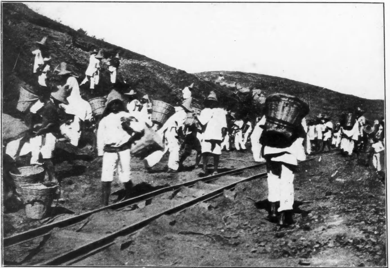
EXCAVATING FOR PINGUICO MILL, GUANAJUATO
