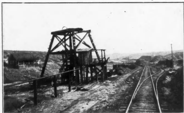
FIG. 3. MCPHERSON SHAFT, USED FOR PROSPECTING PURPOSES
