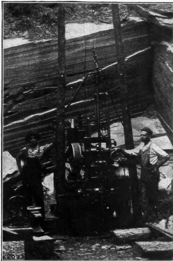
Prospecting with the "Calyx" Drill in a Southern quarry
