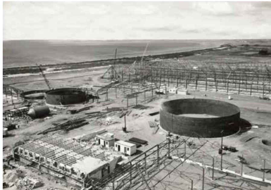
FAR LEFT: Construction offices, March 15, 1962. Photo by Robert Pockley.
