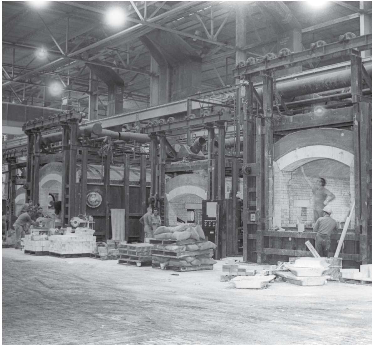
Melting and holding furnaces 5, 6, 7 and 8, Building 810. Photo by K.L. & M. Cecil.
