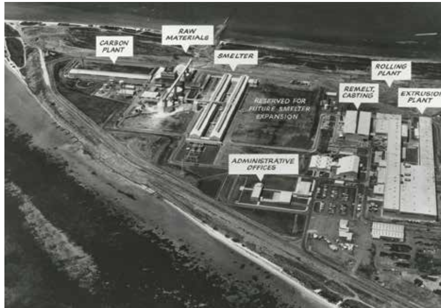
FAR LEFT: Rock and piling for alumina unloading pier, November 11, 1964. Photo by Robert Pockley.
