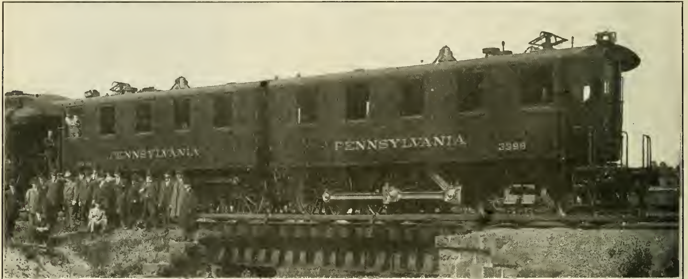
ELECTRIC LOCOMOTIVE FOR HANDLING PENNSYLVANIA RAILROAD TRAINS INTO NEW YORK STATION.
