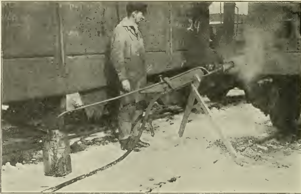
FIG. 20.—CRUDE OIL TORCH FOR HEATING DAMAGED PARTS.
