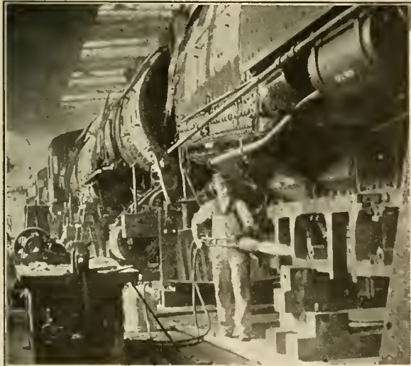
PRE-HEATING A LOCOMOTIVE FRAME.
