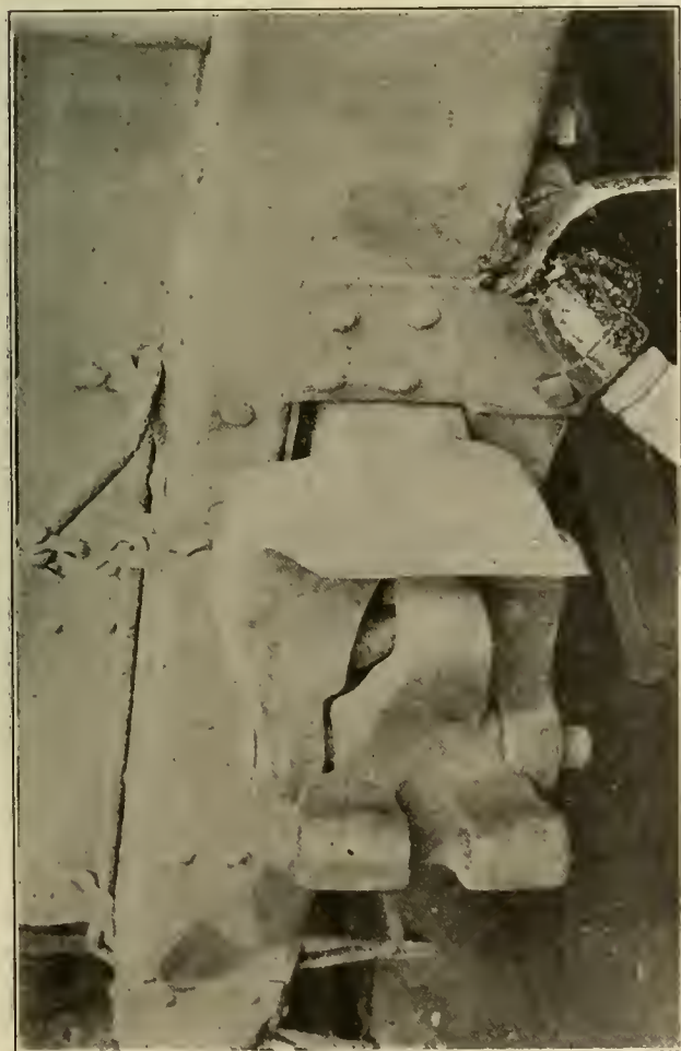
FIG. 32.—END SILL ON G1 HOPPER CAR.
