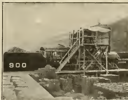
LOCOMOTIVE ARRANGED FOR TESTING SAFETY VALVES.
