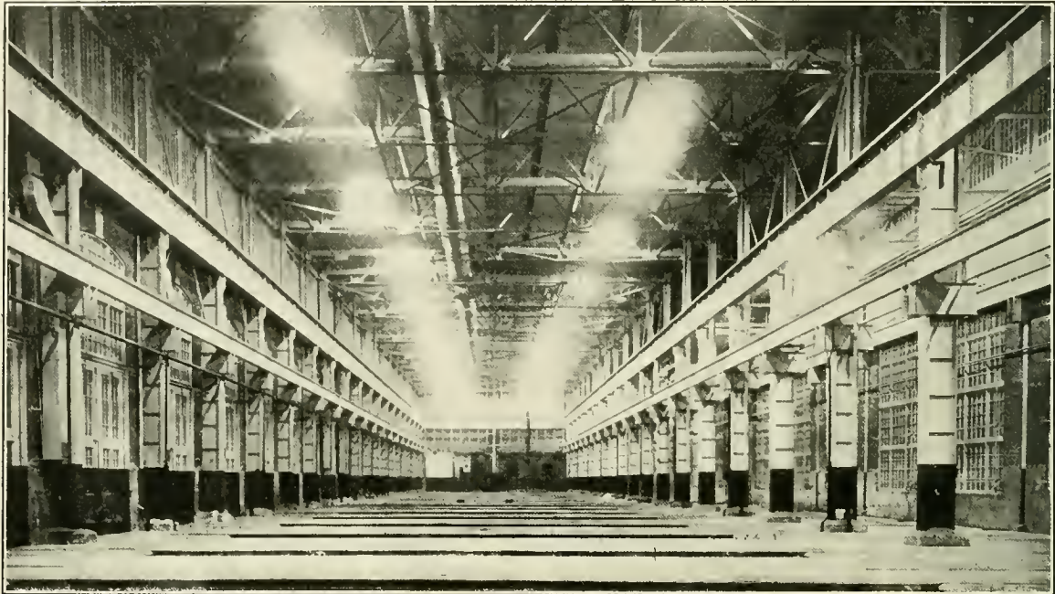
LOCOMOTIVE ERECTING SHOP ILLUMINATED BY COOPER HEWITT LAMPS.
