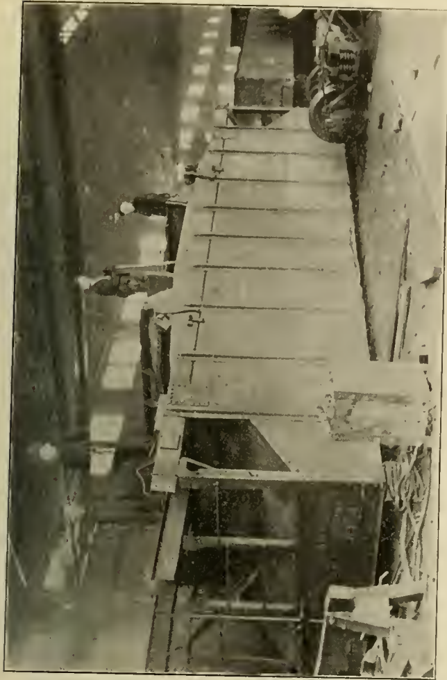
FIG. 14.—HOPPER CAR OVERTURNED AND MEN AT WORK ON CENTER SILLS.
