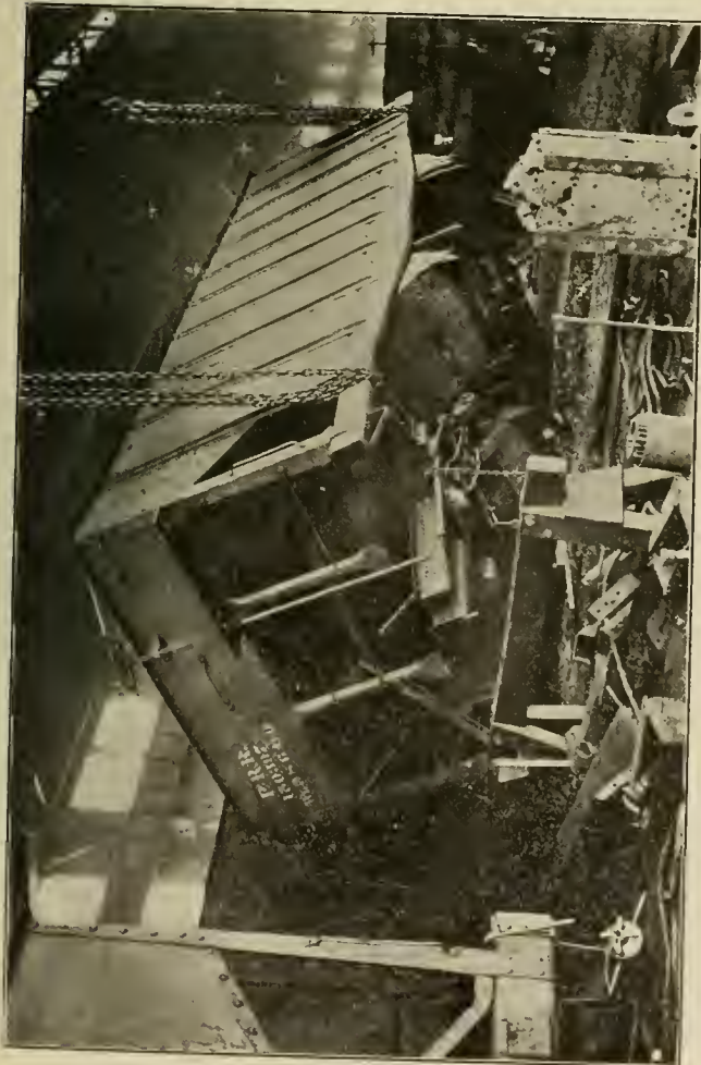
FIG. 12.—FIRST OPERATION IN OVERTURNING A HOPPER CAR IN THE STEEL CAR SHOP.
