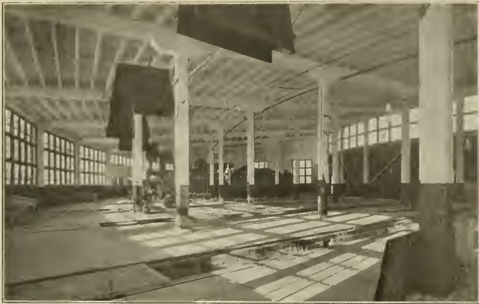
INTERIOR VIEW OF ROUNDHOUSE, IDAHO AND WASHINGTON NORTHERN RY.
