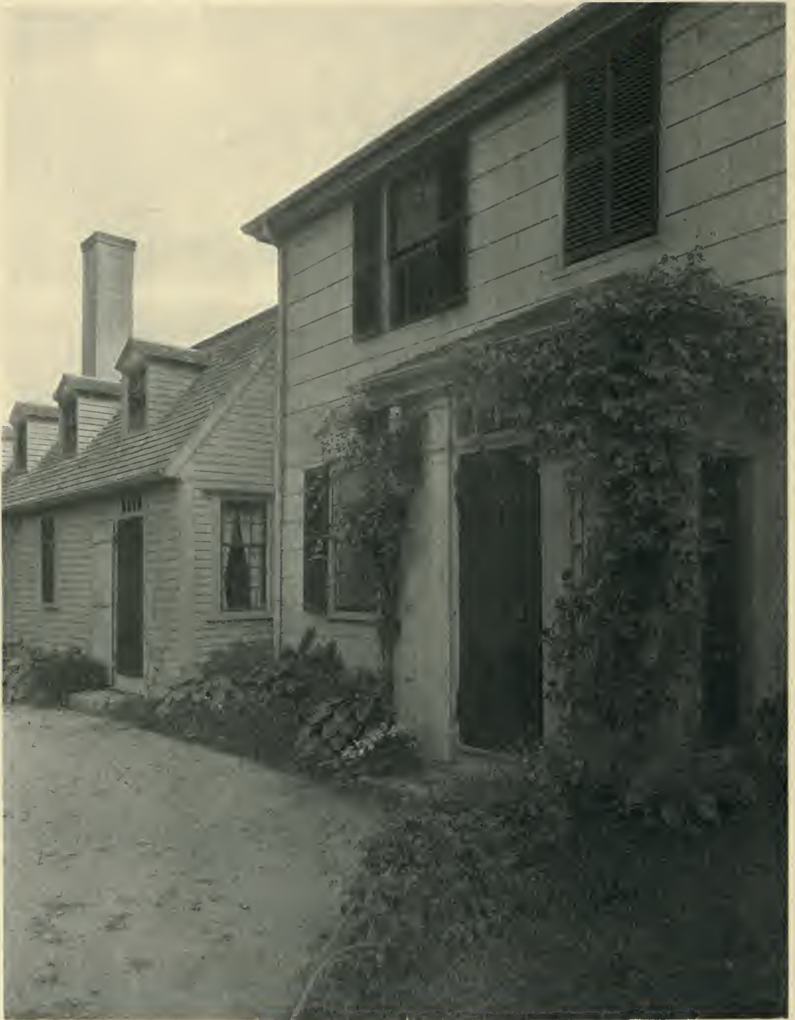
THE SHUTE HOUSE AT HINGHAM, MASS. Detail of Side Entrance
