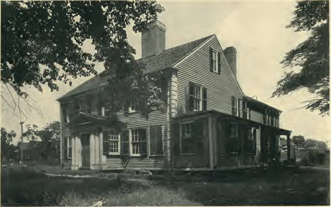
THE OLD BEMIS HOUSE, WATERTOWN, MASS. Built about 1750
