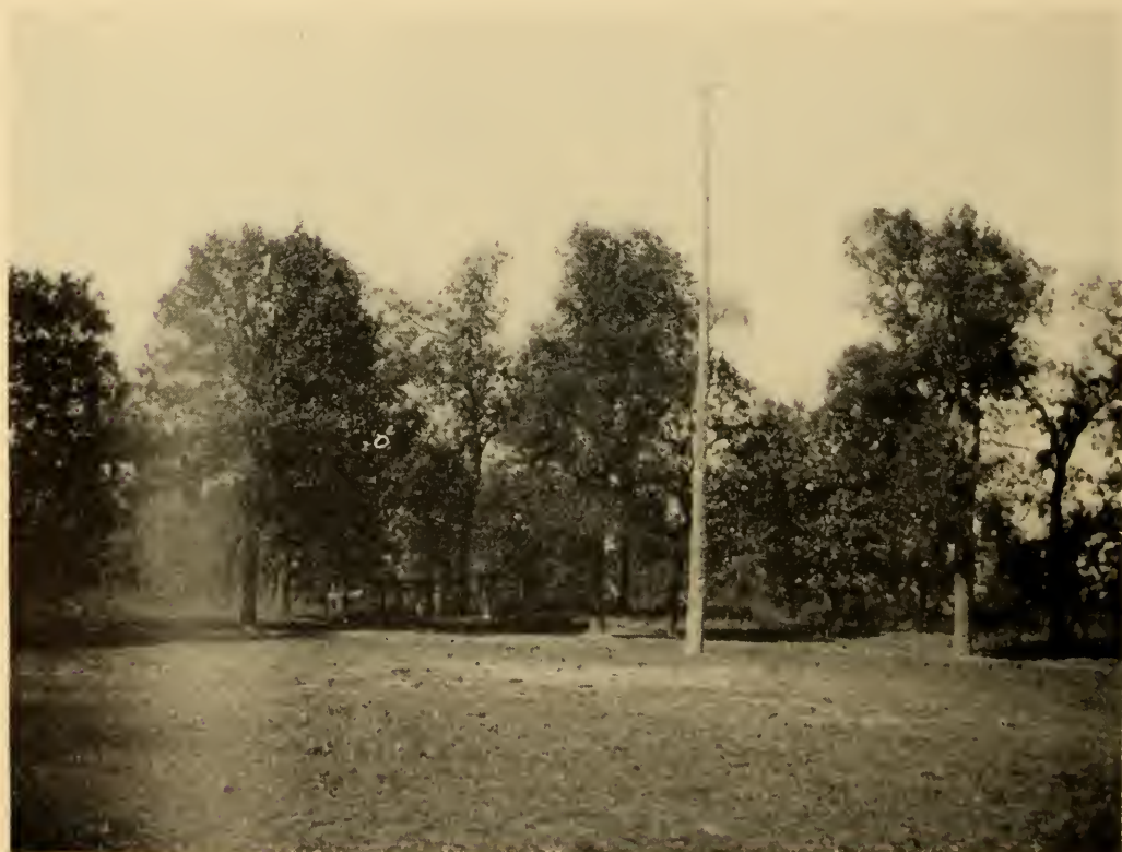
2. BALL POST AND GROUND CONNECTED WITH THE SQUARE GROUND SHOWN ON PLATE 39, FIGURE 2.
