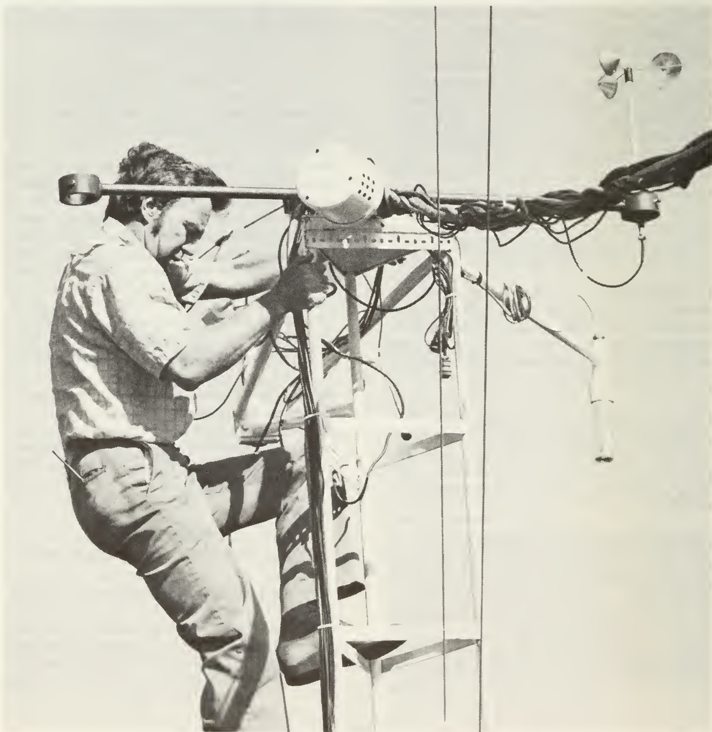
Installing meteorological sensors on the RV/ACANIA
