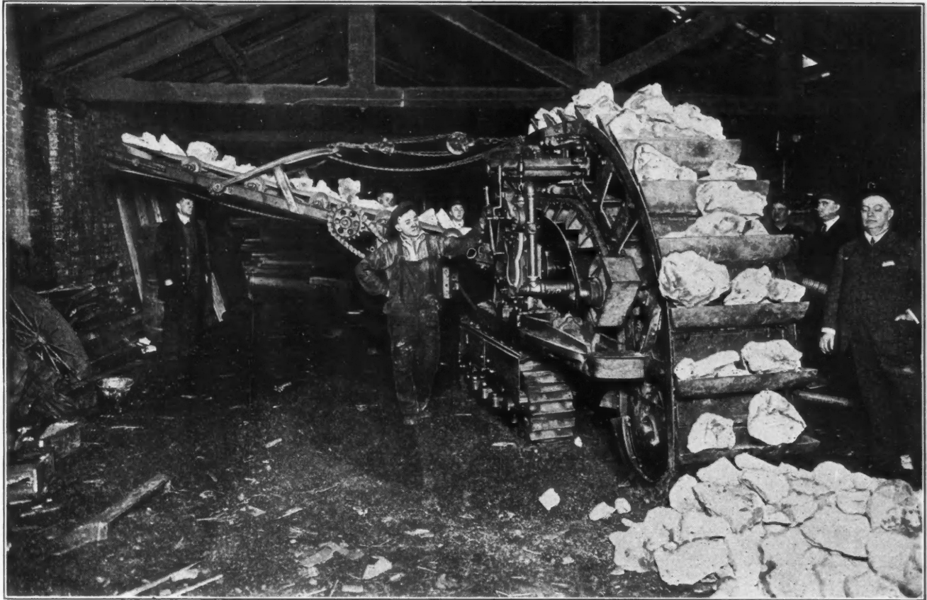
FIG. 12. THE JACKSON SHOVEL WHICH EMBODIES THE BUCKET-ELEVATOR IDEA
