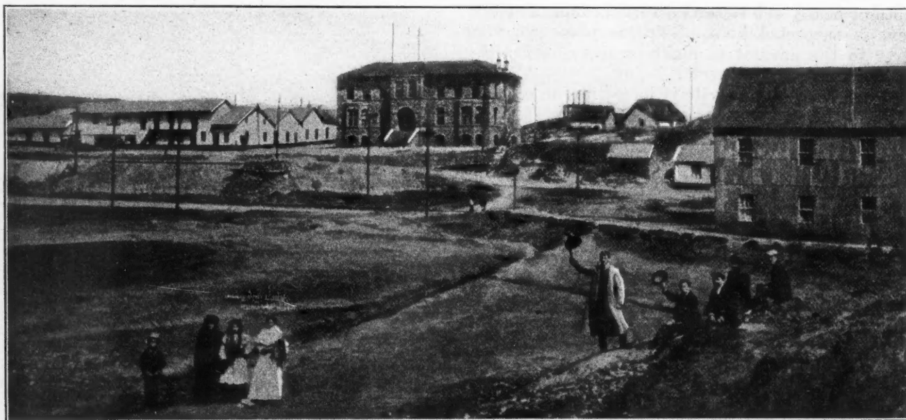
MAIN OFFICE AT CERRO DE PASCO
