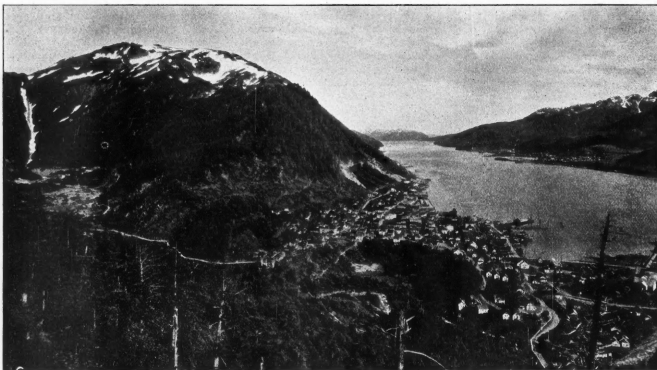
Photo by E. Andrews, Douglas, Alaska ANOTHER VIEW OF JUNEAU, ALASKA, AND GASTINEAU CHANNEL. ON LEFT IS SILVER BOW FAULT. ALASKA JUNEAU MILL IN MIDDLEGROUND ON SLOPE BEYOND TOWN. ORE FROM MINE IS HAULED FROM PORTAL OF TUNNEL AT LEFT OF FAULT AROUND AND THROUGH SHOULDER OF MOUNTAIN AND THENCE TO MILL
