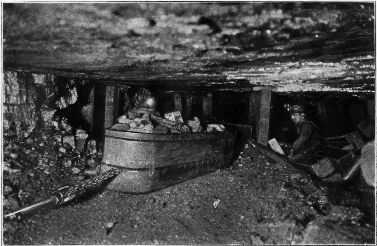
FIG. 48. EVANS SCRAPER IN USE IN A COAL MINE
