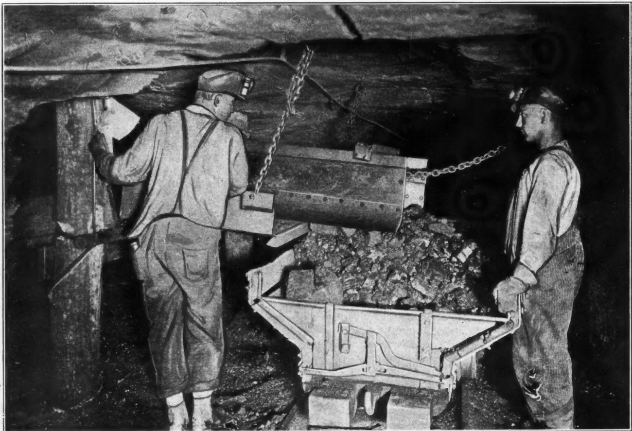
FIG. 49. LOADING TRAM CAR WITH EVANS SCRAPER LOADER
