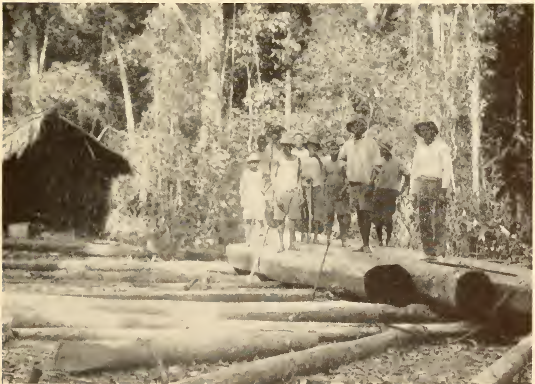
FIG. 58.—Green-heart logs at Lauly's camp on the Upper Pomeroy. These logs are hand-hewn and taken down the river to the saw mill at Pickersgill. Green-heart is used chiefly for piling in docks.
