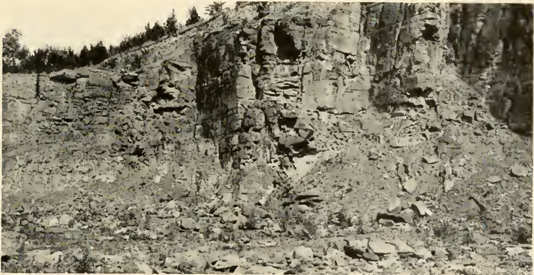
FIG. 16.—Quarry in Stevens Mountain, showing character of Devonian sandstone. From this quarry came most of the rock in Schoharie Reservoir dam.
