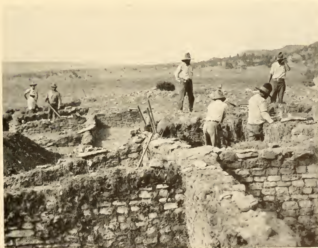
FIG. 160.—Removing débris from the small house.
