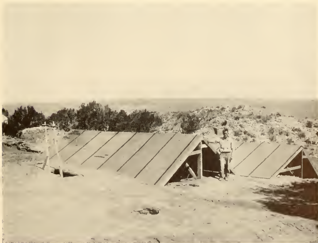
FIG. 142.—Restored pit house in foreground. The shed roofs were erected over other pit remains to preserve them. Large stone mound in background covers ruins of surface house.
