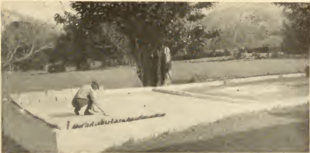
FIG. 64.—A Jamaican "barbecue." Every large estate has one of these concrete platforms for drying coffee and other products.
