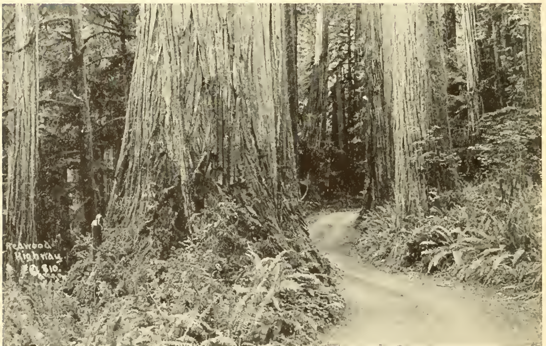
FIG. 94.—Redwood Highway near Smith River, California.
