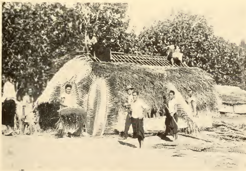
FIG. 68.—Natives roofing a house with the fronds of the cocoanut palm. Very little sugar cane, the leaves of which are generally used by the South Sea Islanders as thatch, is grown on Niuafoou. (Photograph by Kellers.)
