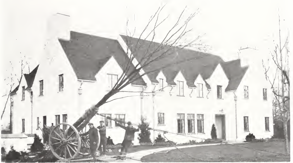
New residence of Adolph Stuber, Esq., Ambassador Drive, Rochester, N. Y. Grading and Seeding—Plans and Planting—Plants and Trees—Wall and Step Construction—photo shows our tree moving crew planting a 12 inch Elm selected at Glenwood Nursery. Entire job by Glen Brothers, Inc., Landscape Dept.
