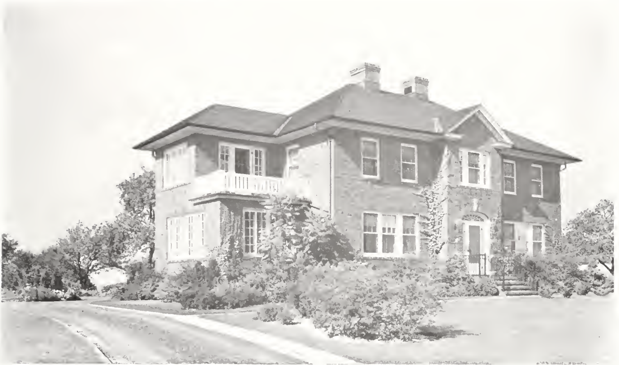
Home of Mr. A. J. Mathews, Potsdam, N. Y. Plans, Plants, Planting, Glen Bros. Inc. Landscape Dept. Rochester, N. Y.
