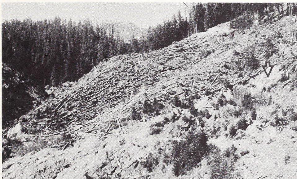
Figure 88. Ground photo of the new slump outlined in Figure 87. The arrow indicates ground water seeping from the face of the scarp.
