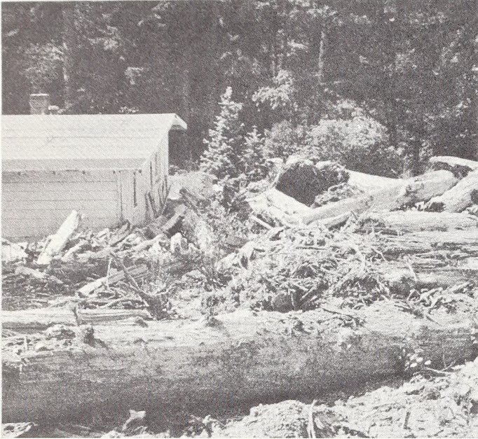
Figure 56. The result of a debris avalanche from a road fill in a headwall in sandstone material
