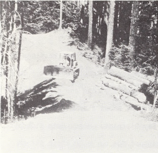
Figure 61. Endhailed material may be compacted on flattened ridges.
