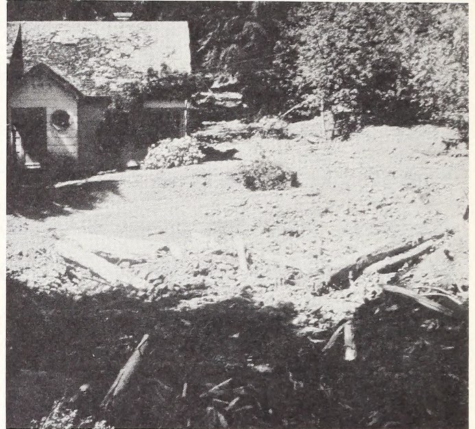
Figure 57. A debris flow came down the stream channel just to the right of the house
