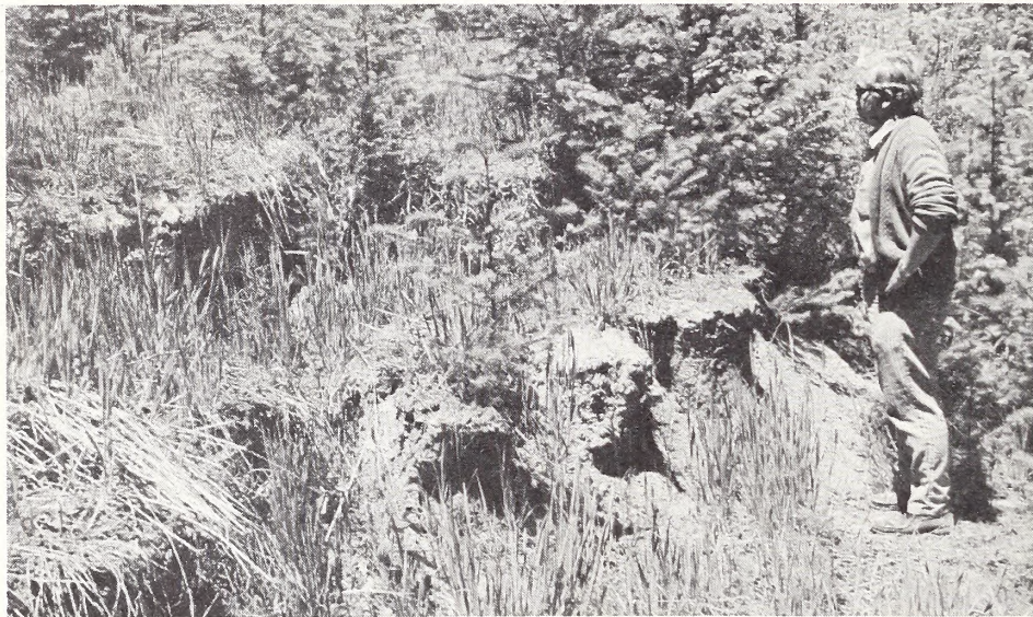
Figure 67. Cat steps, or small scarps, result from slope failures.
