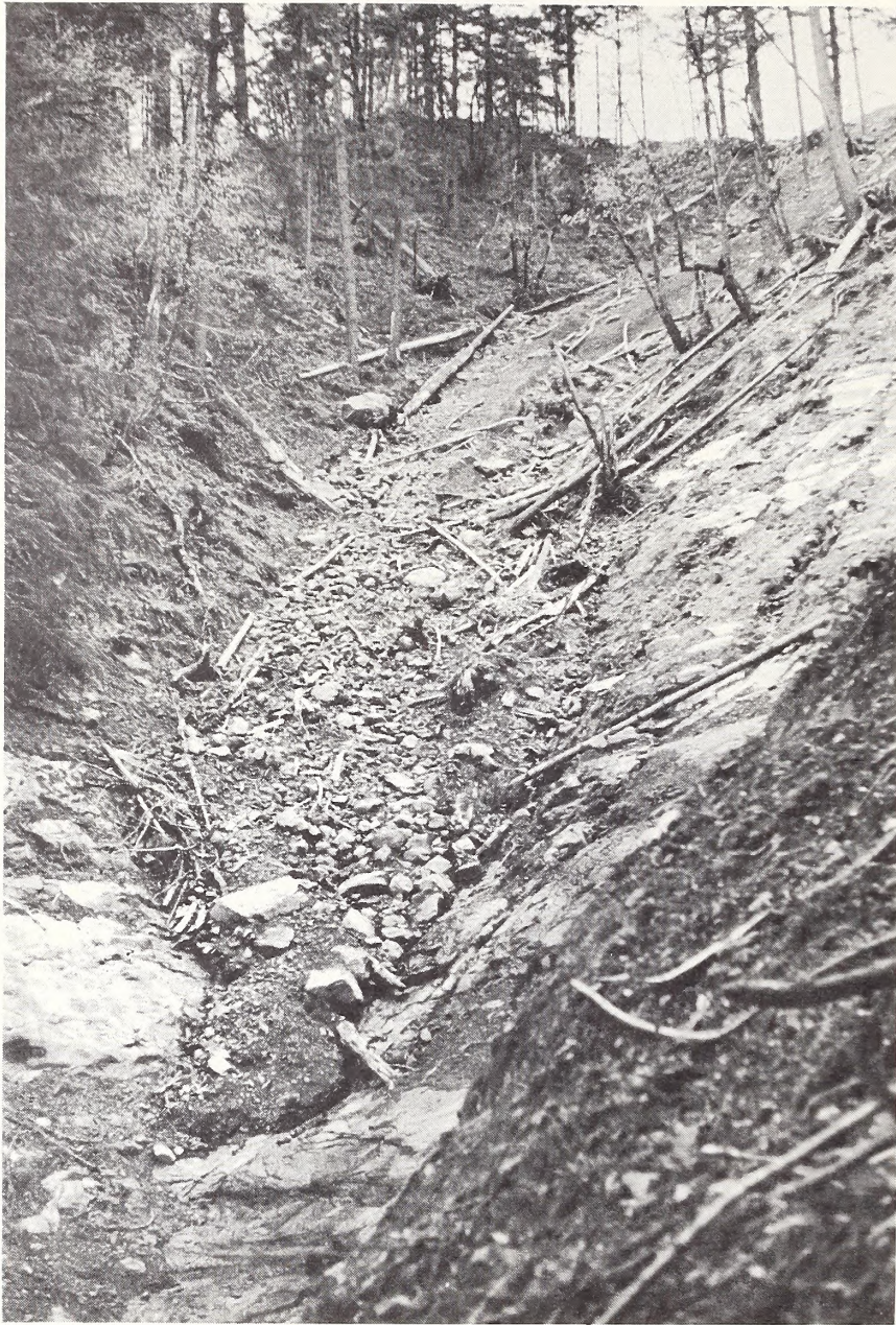
Figure 104. Rubble from road clearance has been deposited in this steep headwall. This increases the potential for another slide.
