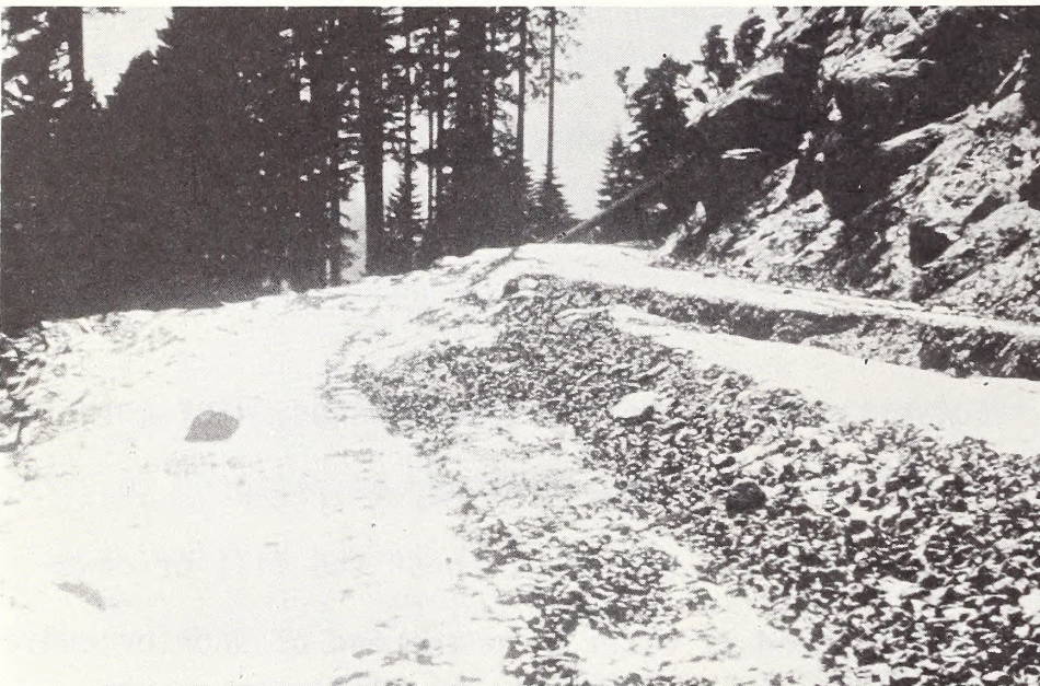
Figure 61. Endhailed material may be compacted on flattened ridges.
