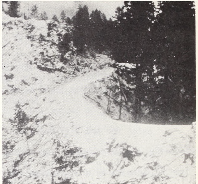
Figure 62. This ridge road has remained stable for two winters.
