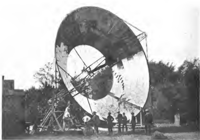
New Solar Motor erected near Boston
