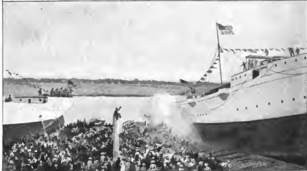
Launching a Ship from the Slips of One of the Largest Ship-building Companies in the World
