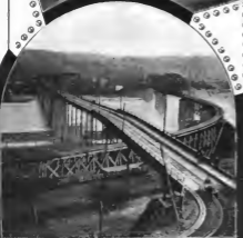
HIGHWAY BRIDGE OVER MONONGAHELA RIVER, MCKEESPORT, PA.
