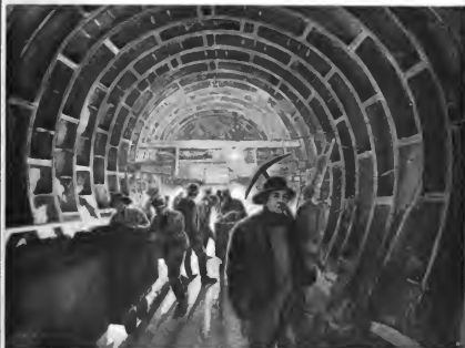
Working on the Tunnel in the Compressed-air Shaft
