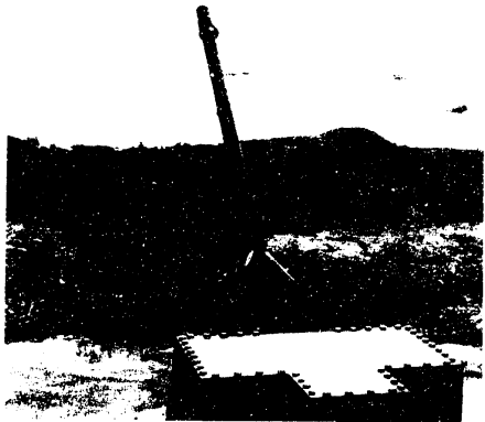
FIGURE 23. Fixed coastal artillery battery (U/OU)
