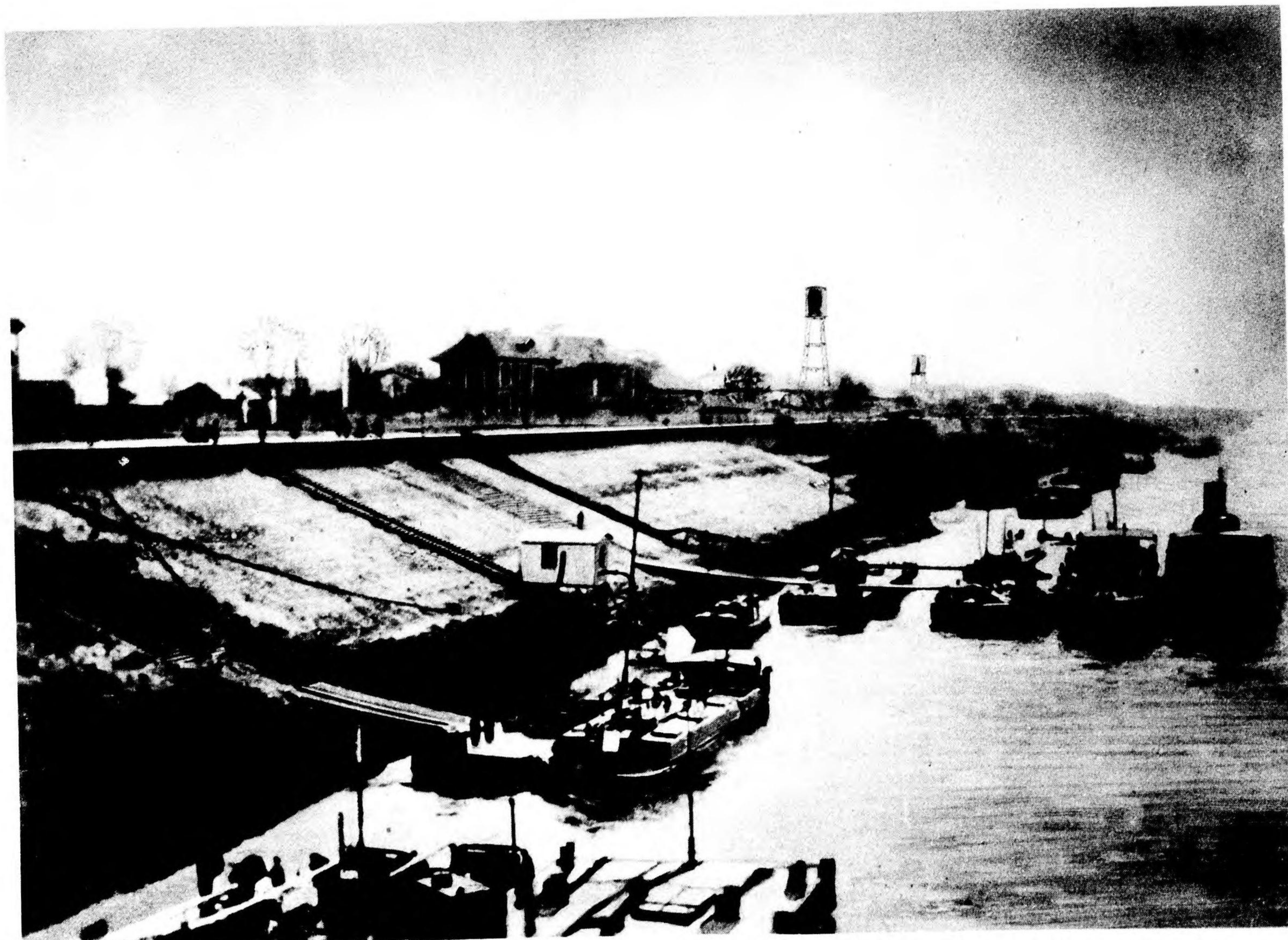
WATER FRONT VIEW OF ASIATIC PETROLEUM CO. AND STANDARD-VACUUM OIL CO. INSTALLATIONS AT HANKOW, SHOWING RIVER BANK STEPS, MOVABLE PUMPHOUSES AND HOSE CONNECTIONS
