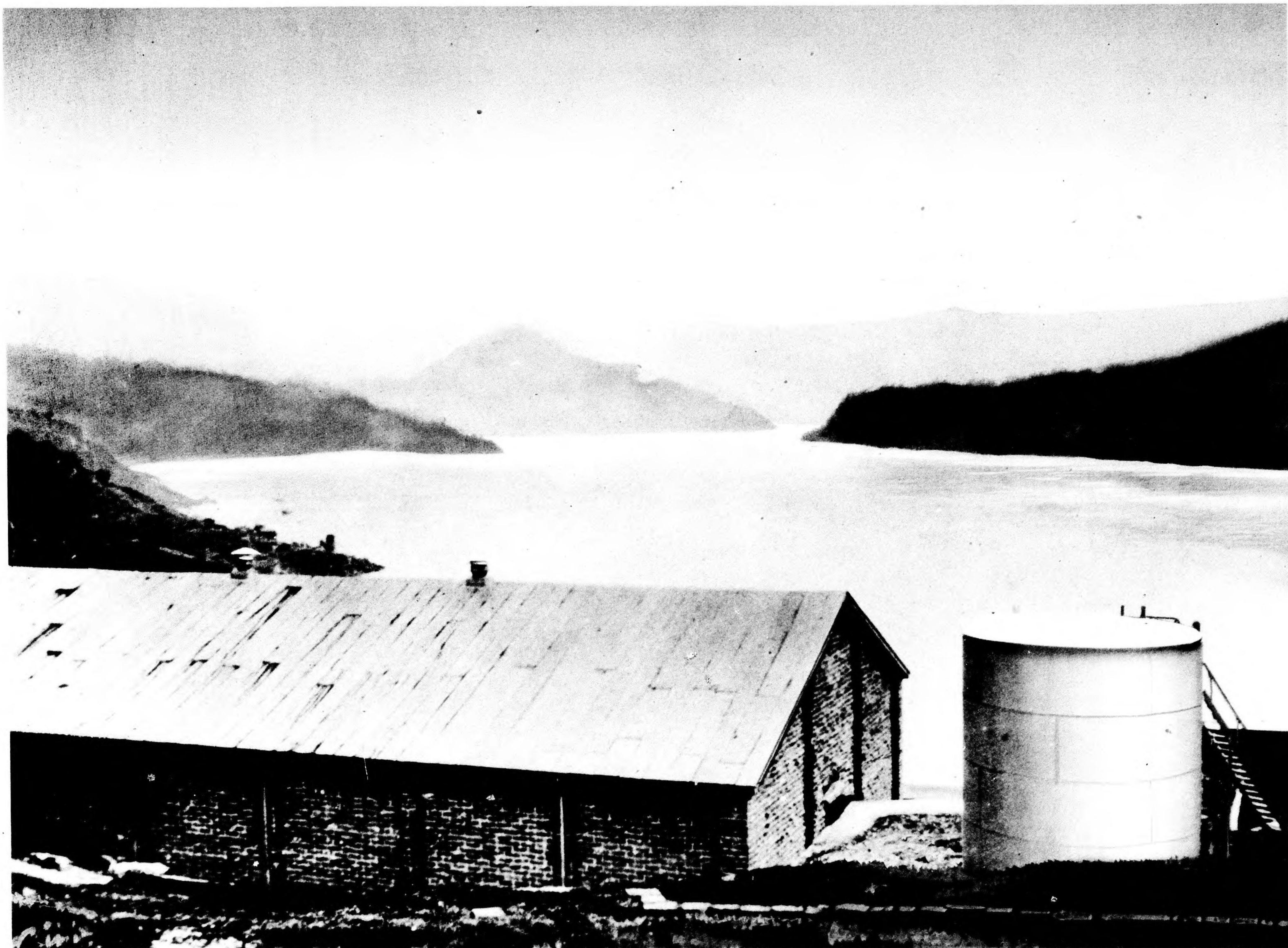
STANDARD-VACUUM OIL CO. WANHSIEN INSTALLATION
