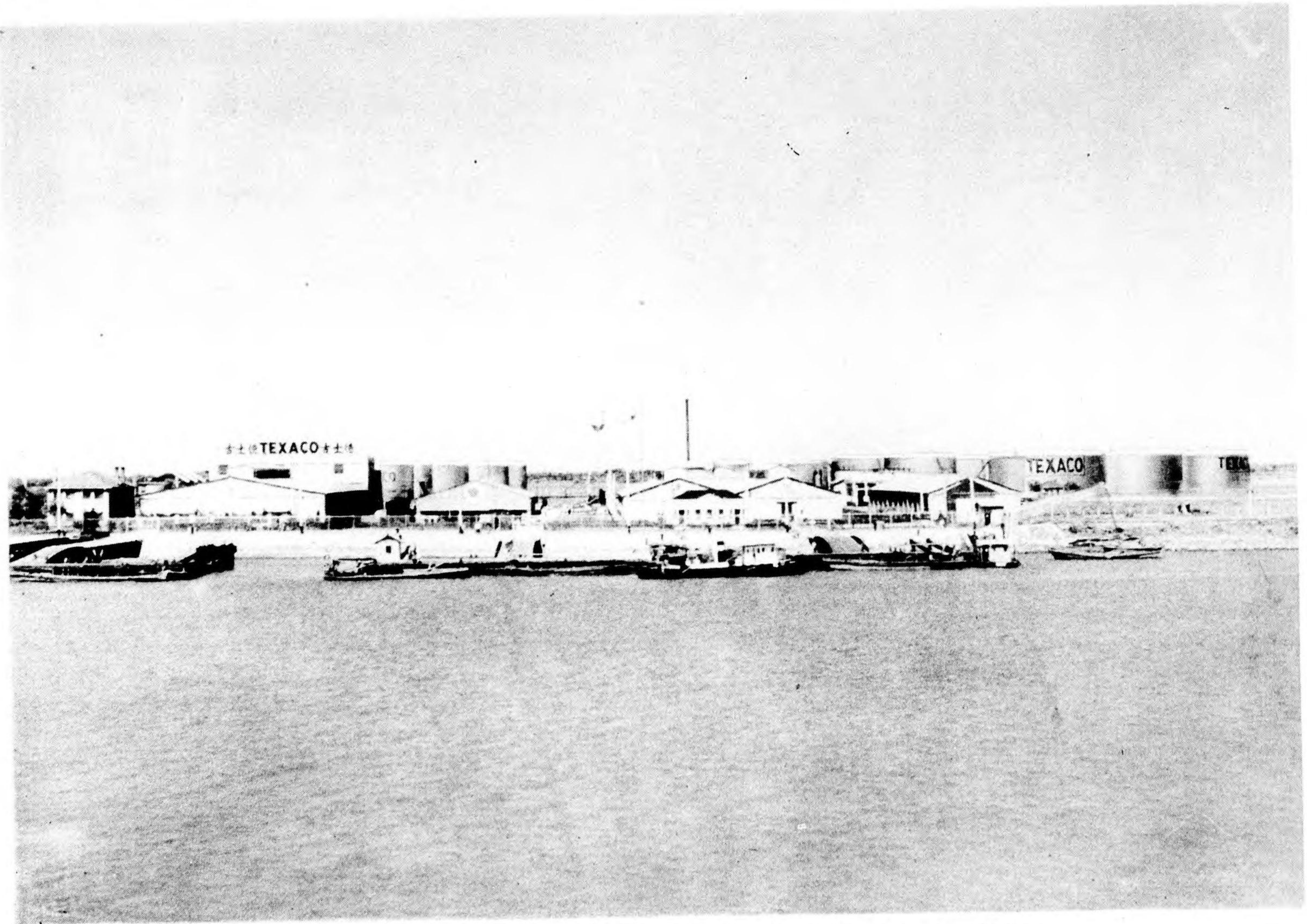
TWO VIEWS OF THE TEXAS CO. GOUGH ISLAND INSTALLATION, SHANGHAI
