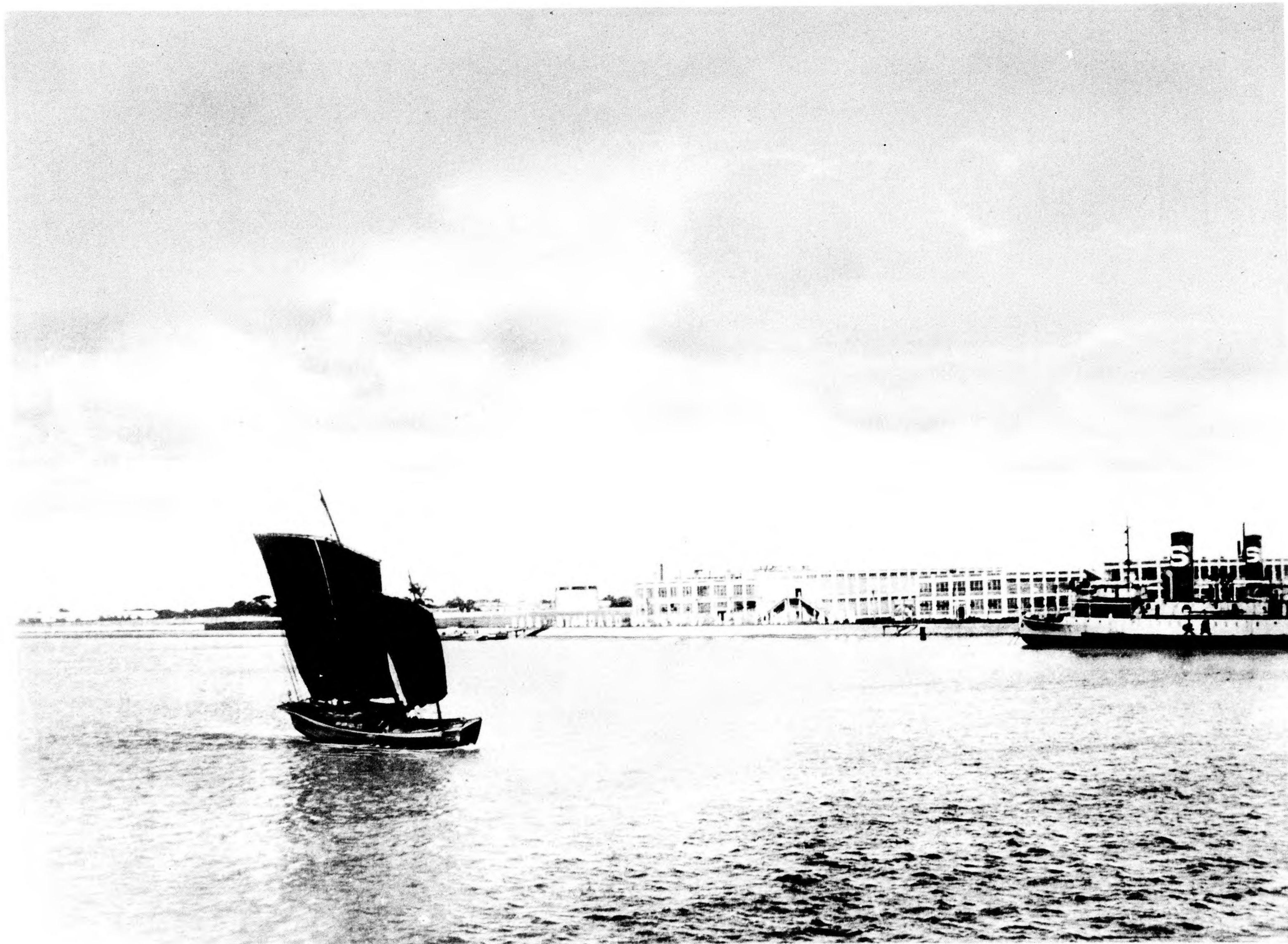
LOWER PART OF STANDARD-VACUUM OIL CO. POOTUNG INSTALLATION SHOWING MACHINE SHOP AND GASOMETER TANK FOR AVIATION GASOLINE STORAGE
